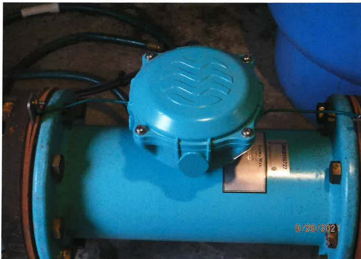
FLOW METER INSTALLED FROM 15,000 GAL STORAGE TANK TO USES
