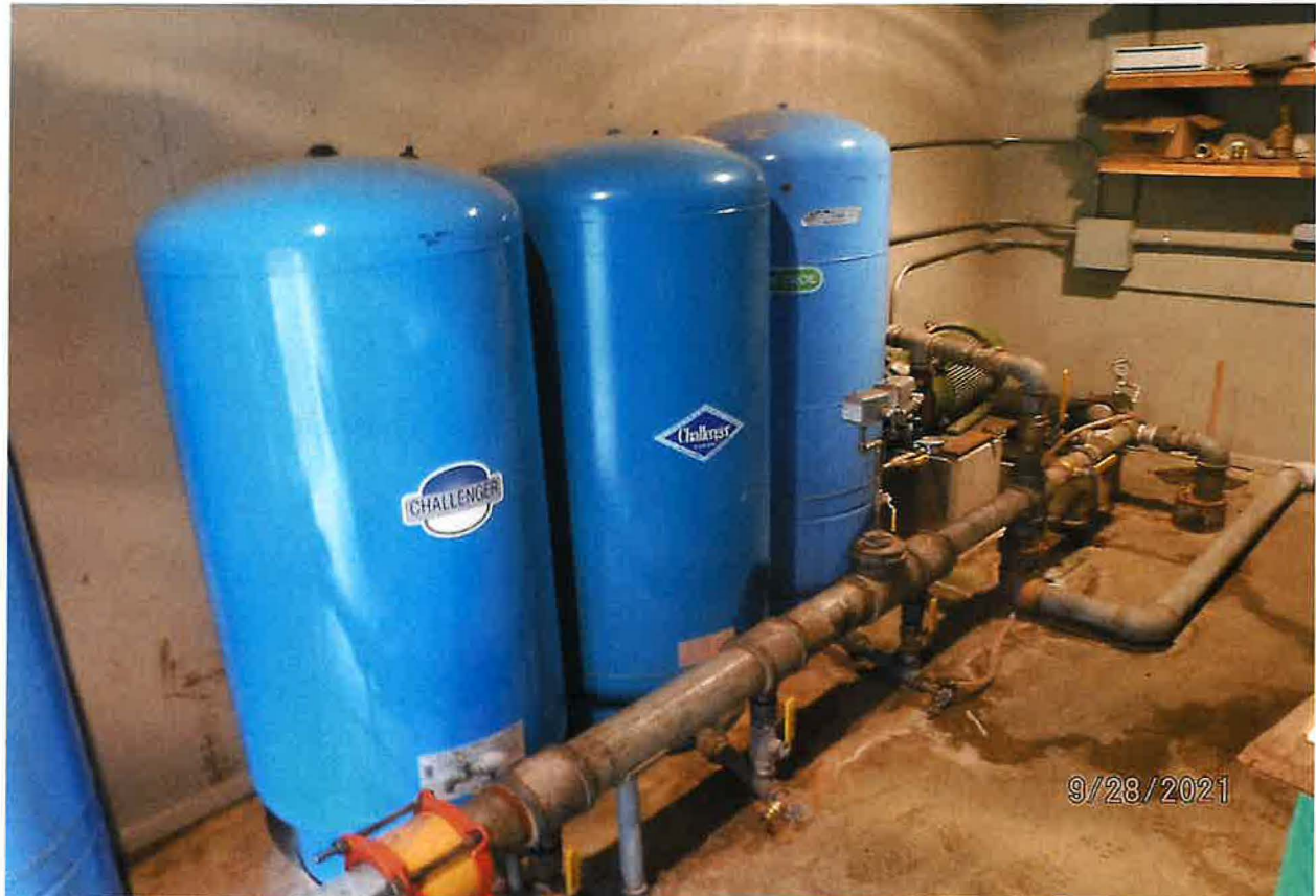
WATER SYSTEM DIVERTING WORKS
