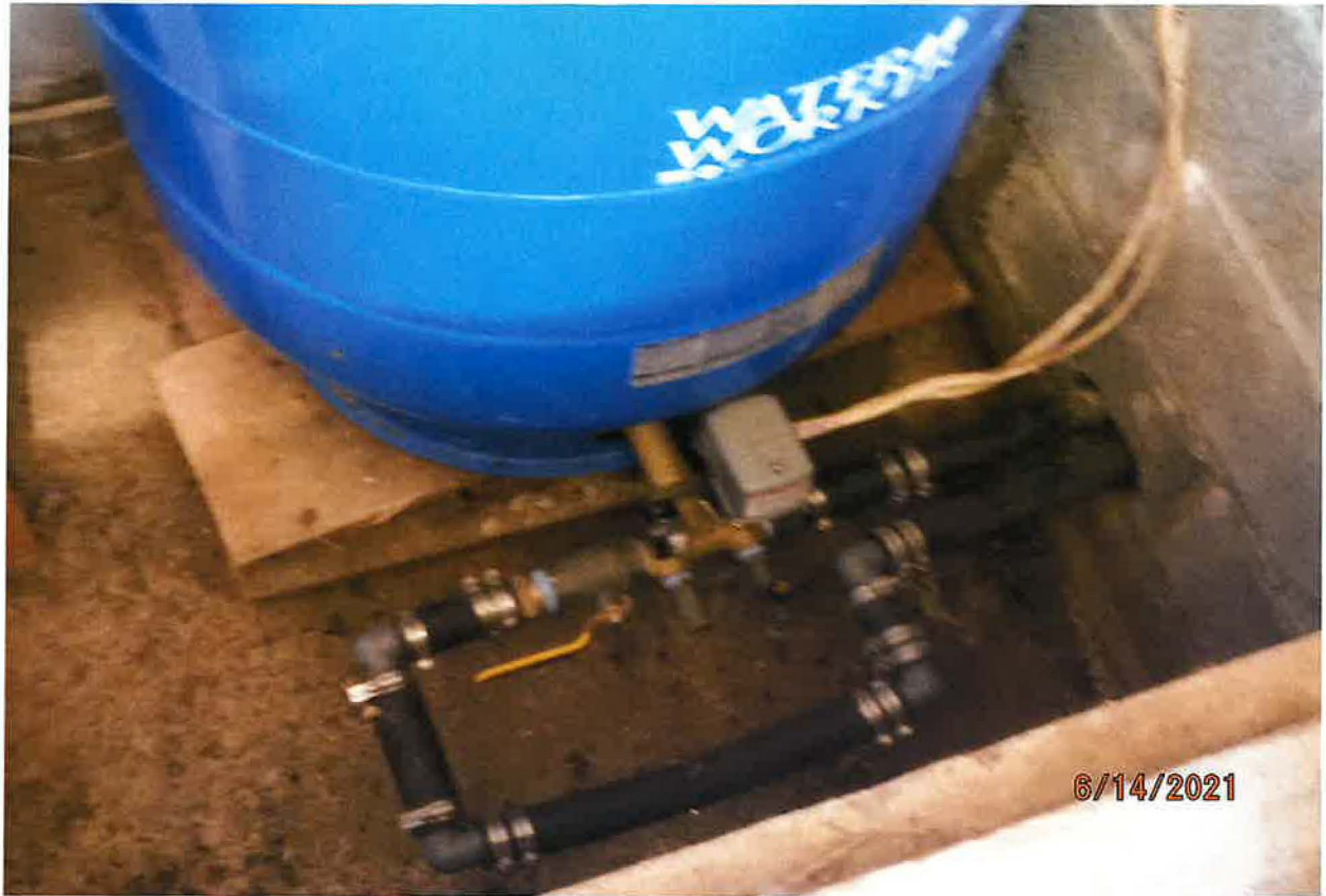
WATER CONVEYANCE SYSTEM
