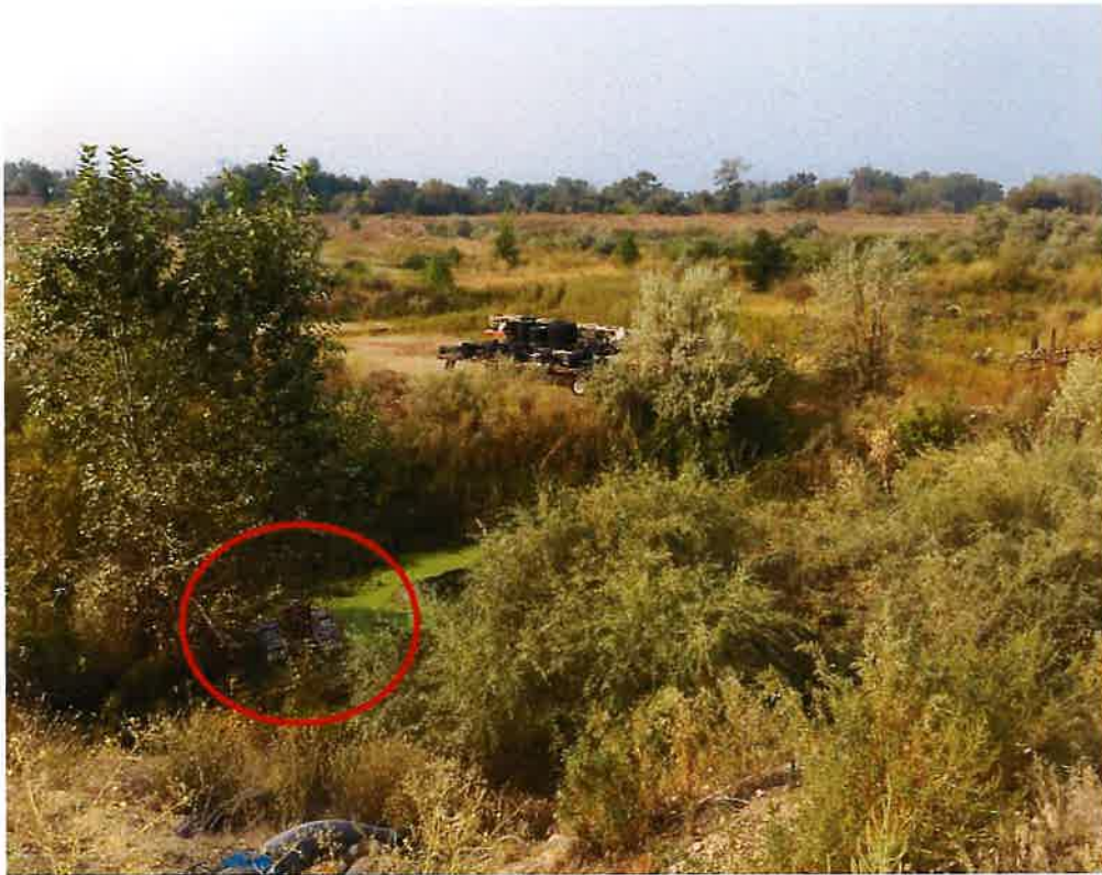
Figure 3: Pump dewatering pit near the discharge pipe (POD)
