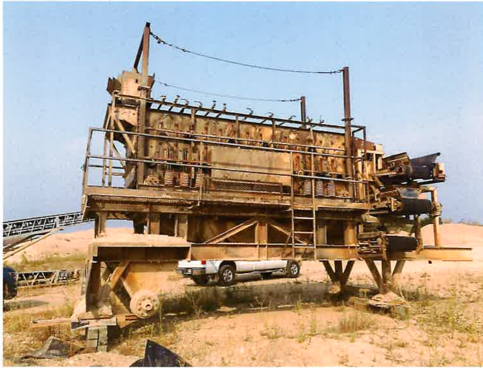
Figure 5: Part of the crusher/wash plant that currently is not being used.
