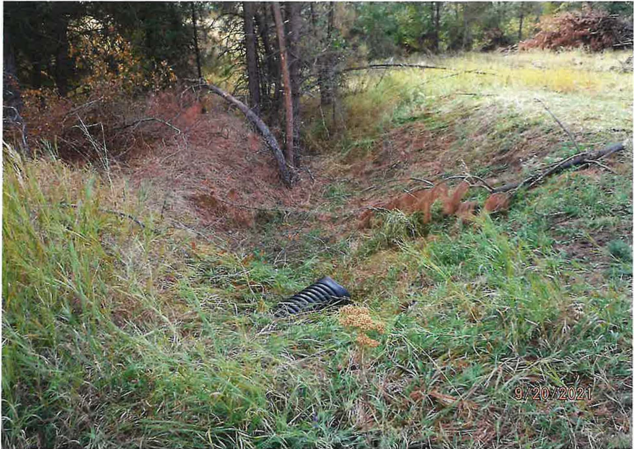
NORTHERN POND OVERFLOW DEVICE OUTFLOW CHANNEL W/PIPE
