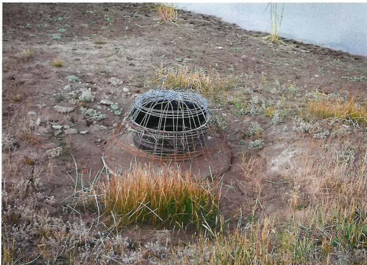
SOUTHERN POND – OVERFLOW DEVICE & ROCK CHANNEL
