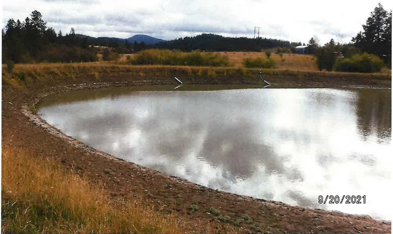
POD – SOUTHERN POND DAM
