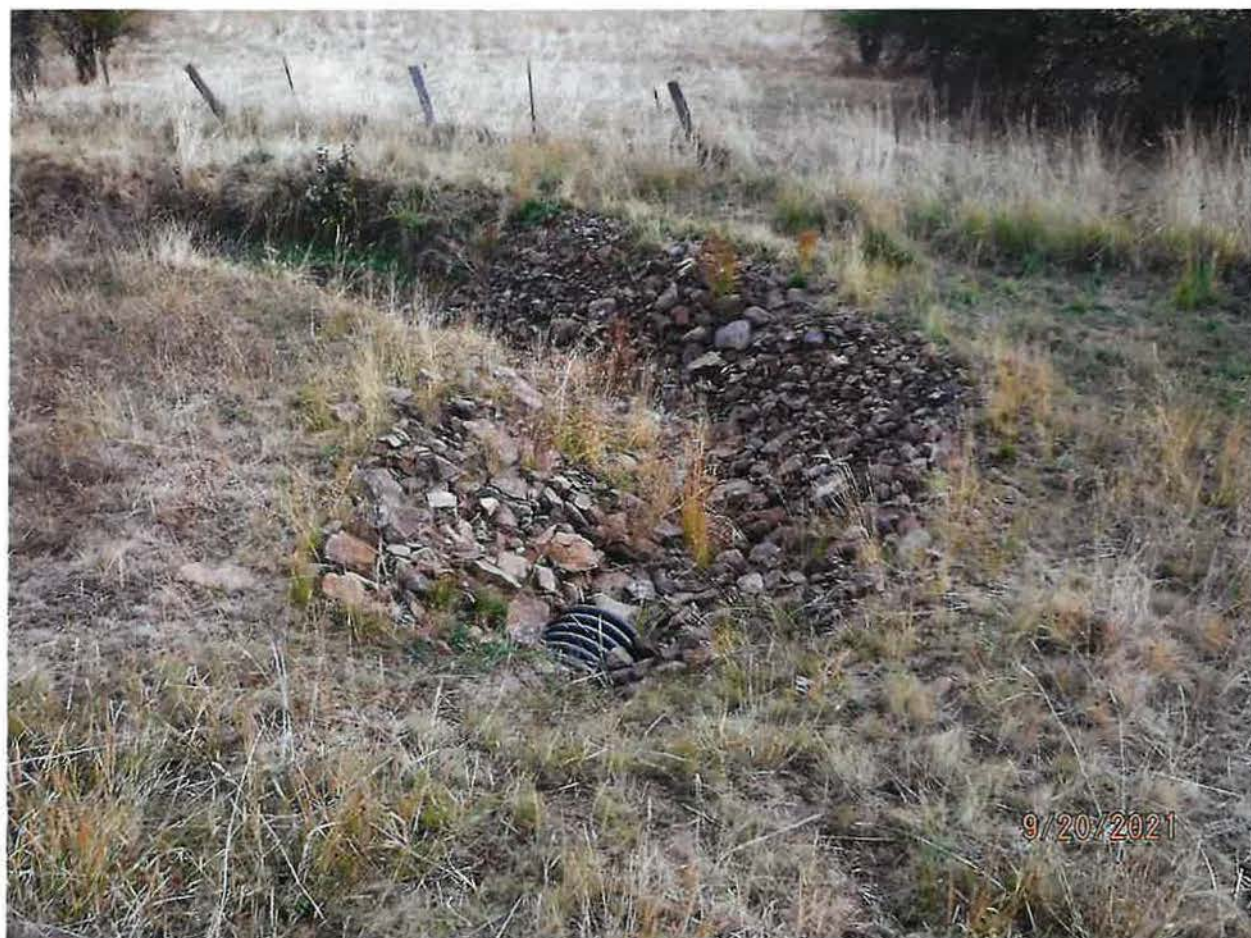
SOUTHERN POND – OVERFLOW DEVICE & ROCK CHANNEL
