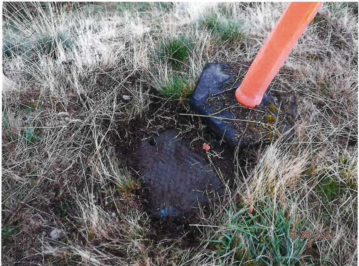
IRRIGATION POU – EXAMPLE PRESSURIZED IRRIGATION VALVE SPLITTER STATION
