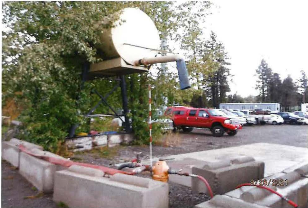
INDUSTRIAL POU - WATER TRUCK FILL STATION – CO-LOCATED WITH 30K STORAGE RESERVOIR
