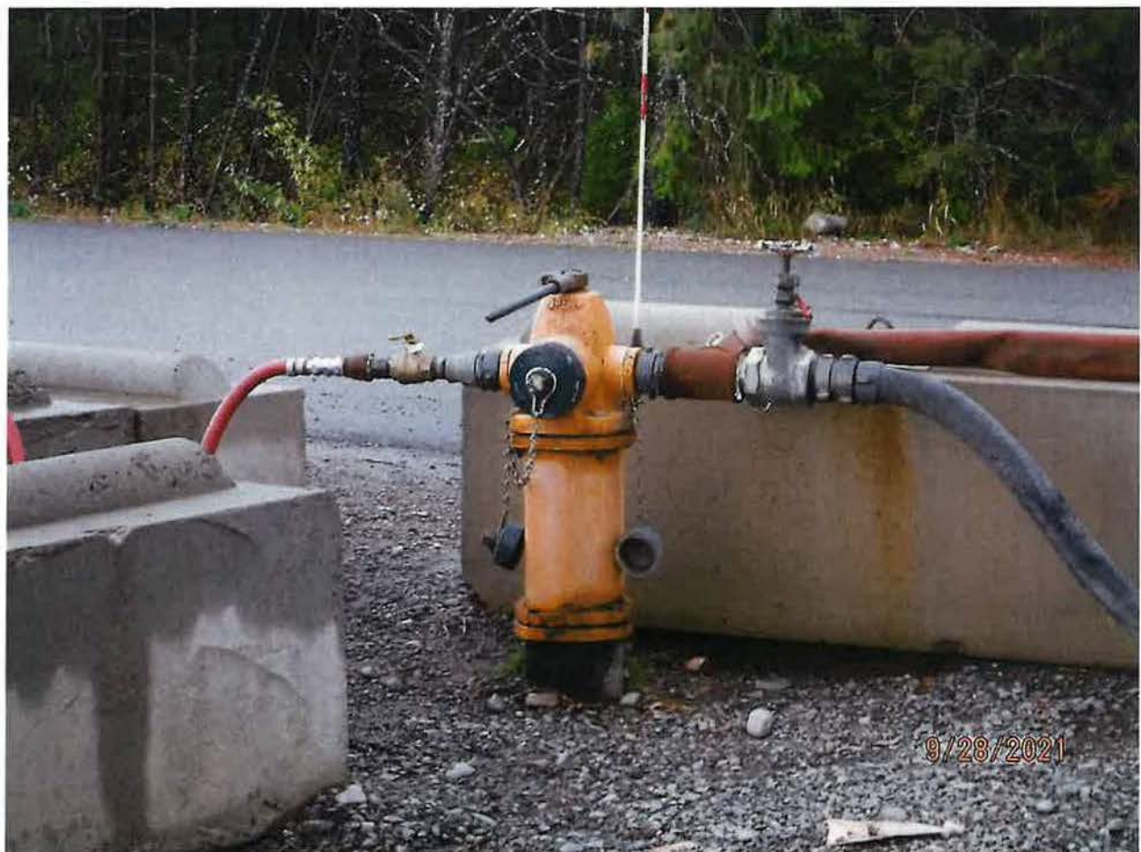
INDUSTRIAL POU - WATER TRUCK FILL STATION – CO-LOCATED WITH 30K STORAGE RESERVOIR
