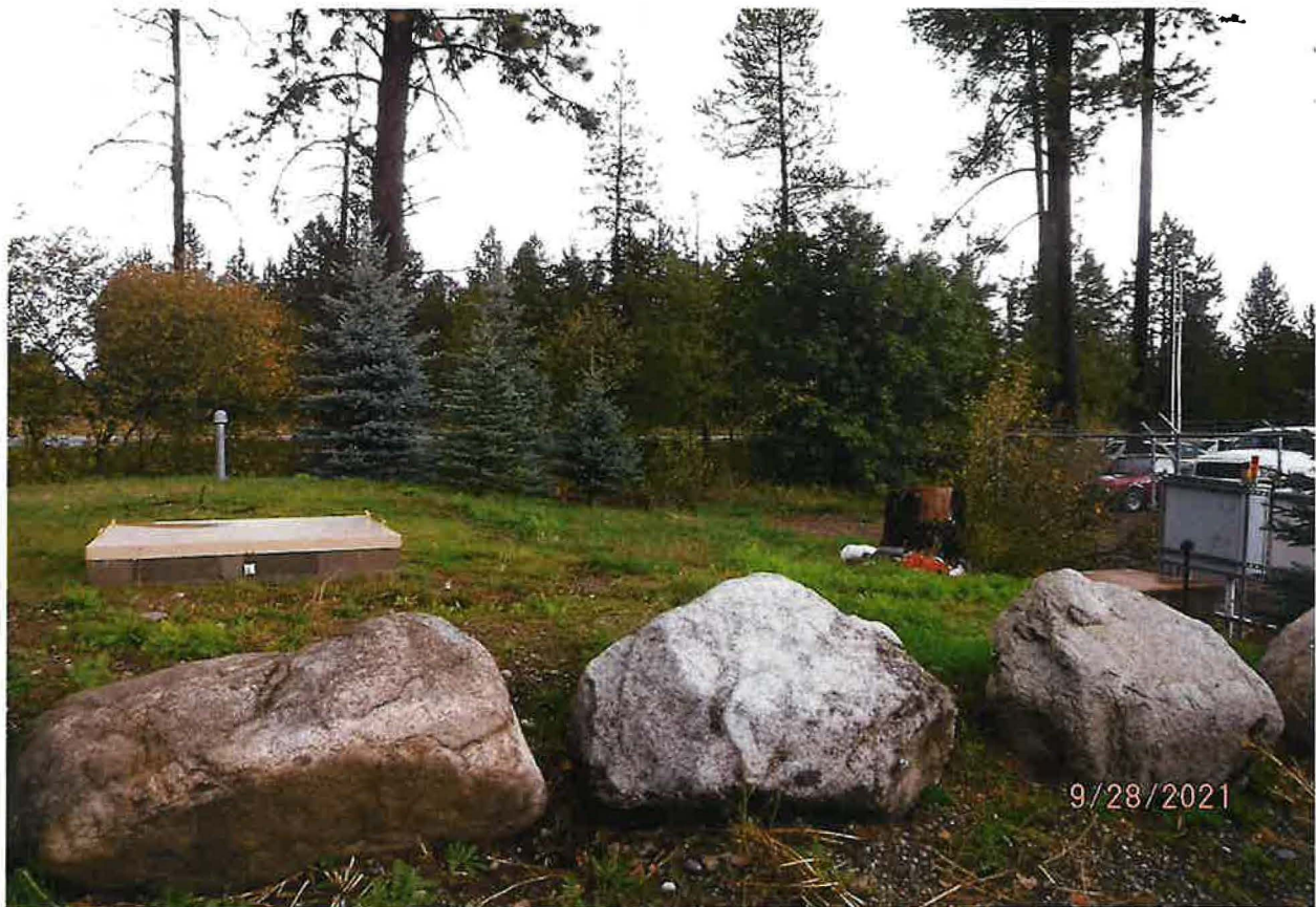
VAULTED DIVERSION WORKS (R/H OF IMAGE METAL LID)
