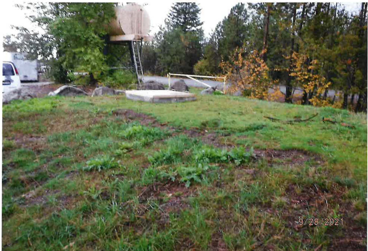
30,000-GAL VAULTED STORAGE RESERVOIR
