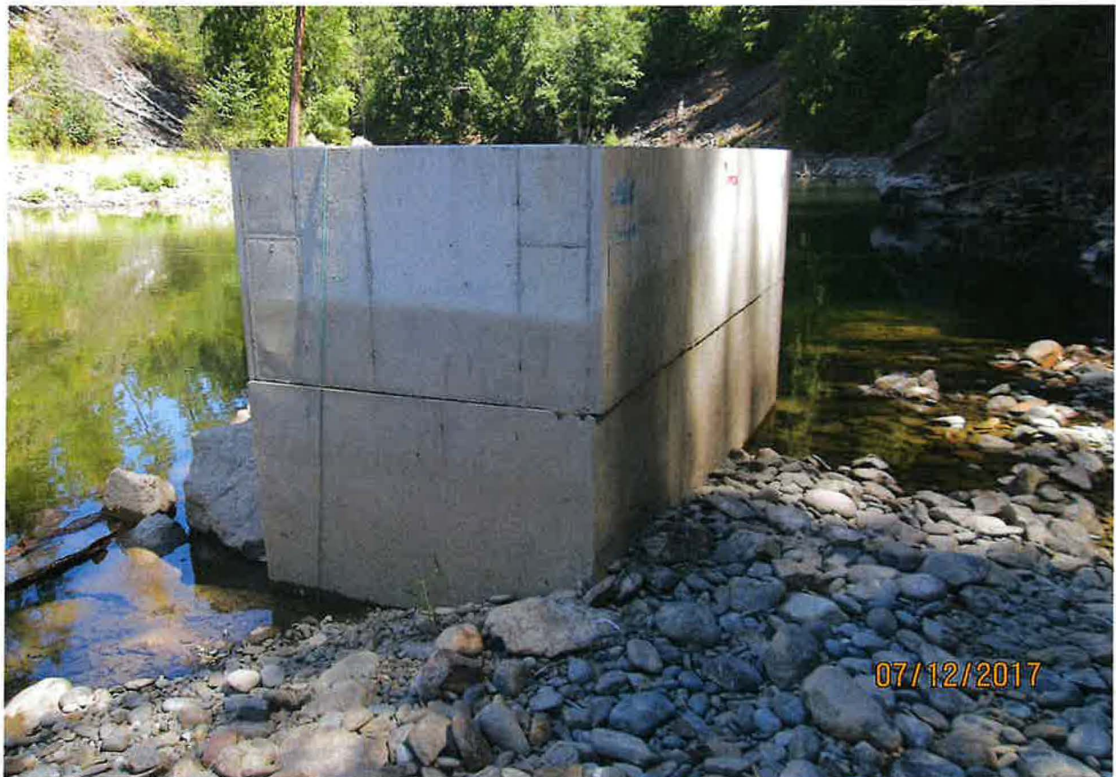
POD – MOYIE RIVER INTAKE WORKS
