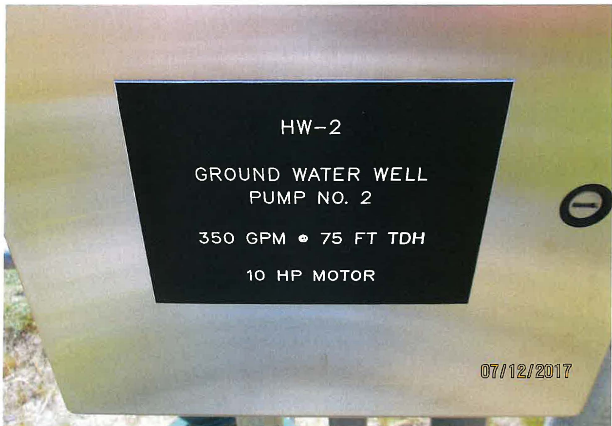
POD – D0058065 – 10 HP MOTOR INSTALLED
