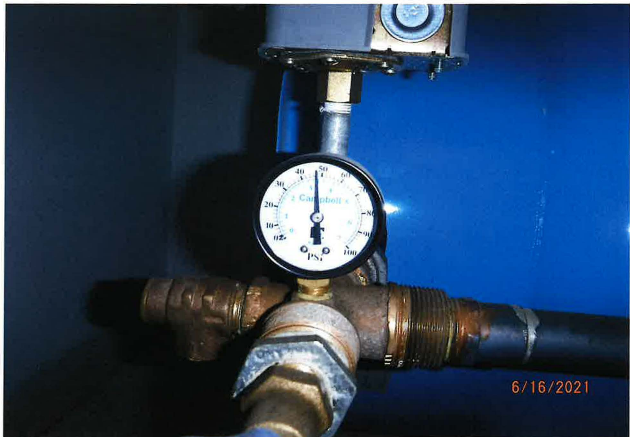
45 – 48 PSI SYSTEM OPERATING PRESSURE
