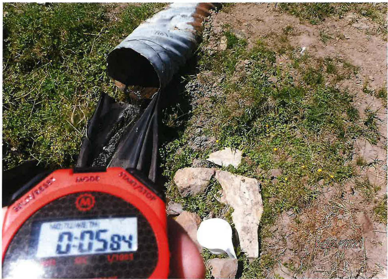
4-CUP MEASURING DEVICE USED AT CULVERT TO CAPTURE DIVERSION RATE
