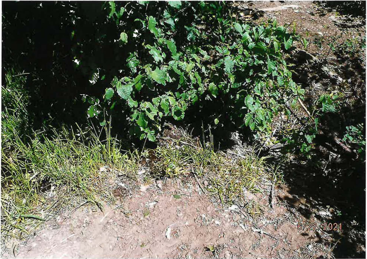
POD – EARTHEN DAM WITH OVERFLOW CHANNEL FROM SMALL POND
