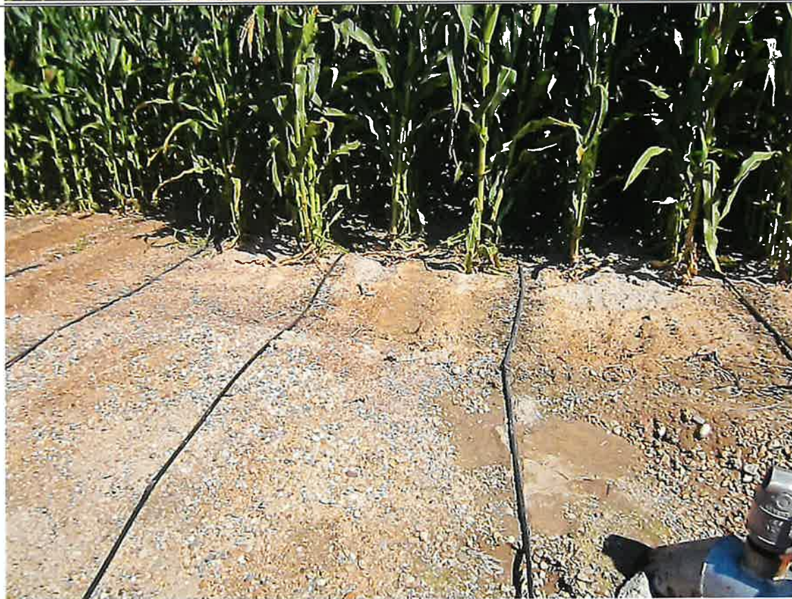
Figure 12. Driplines irrigating pivot corners on 79 acre 63-11615 POU.
