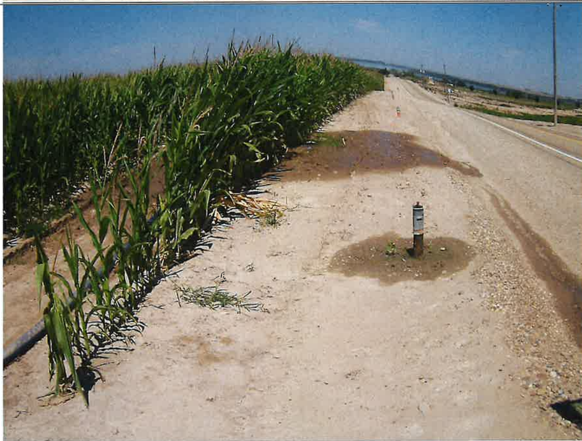
Figure 10. Remanent risers along Farmers Road. This mainline conveys water to 63-33744 POU.
