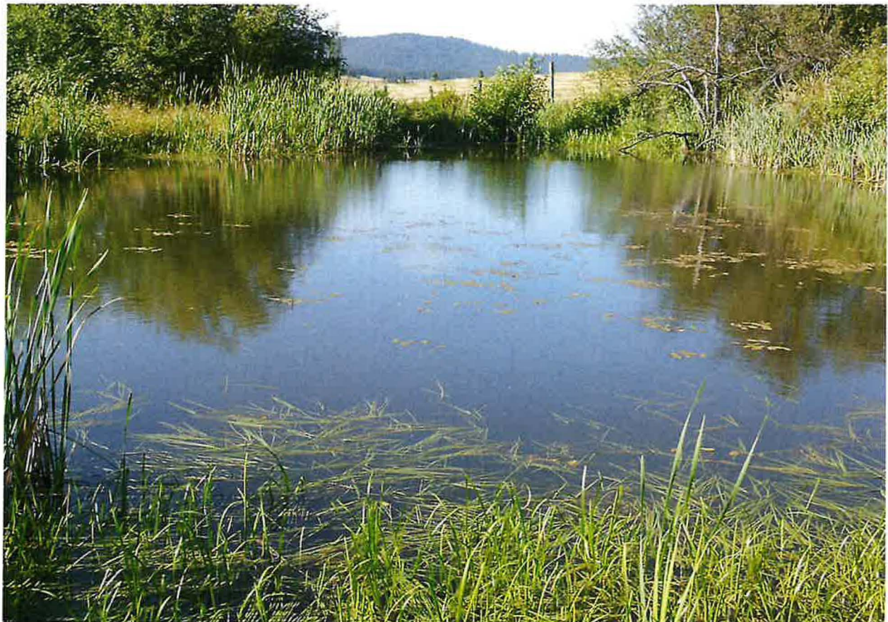
POND POD – EARTHEN DAM WITH OVERFLOW PIPE
