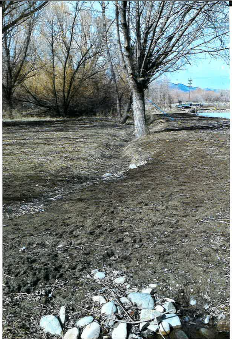
Overflow Ditch- Flows to the side of the pond & converges with pond water over/past the pond gate.
