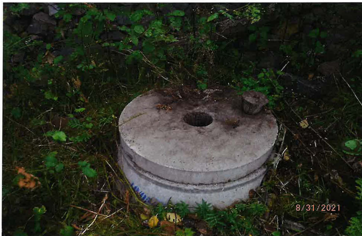
POD – SPRING FLOW TO CONCRETE CISTERN (SAME POD AS WR 96-9615)
