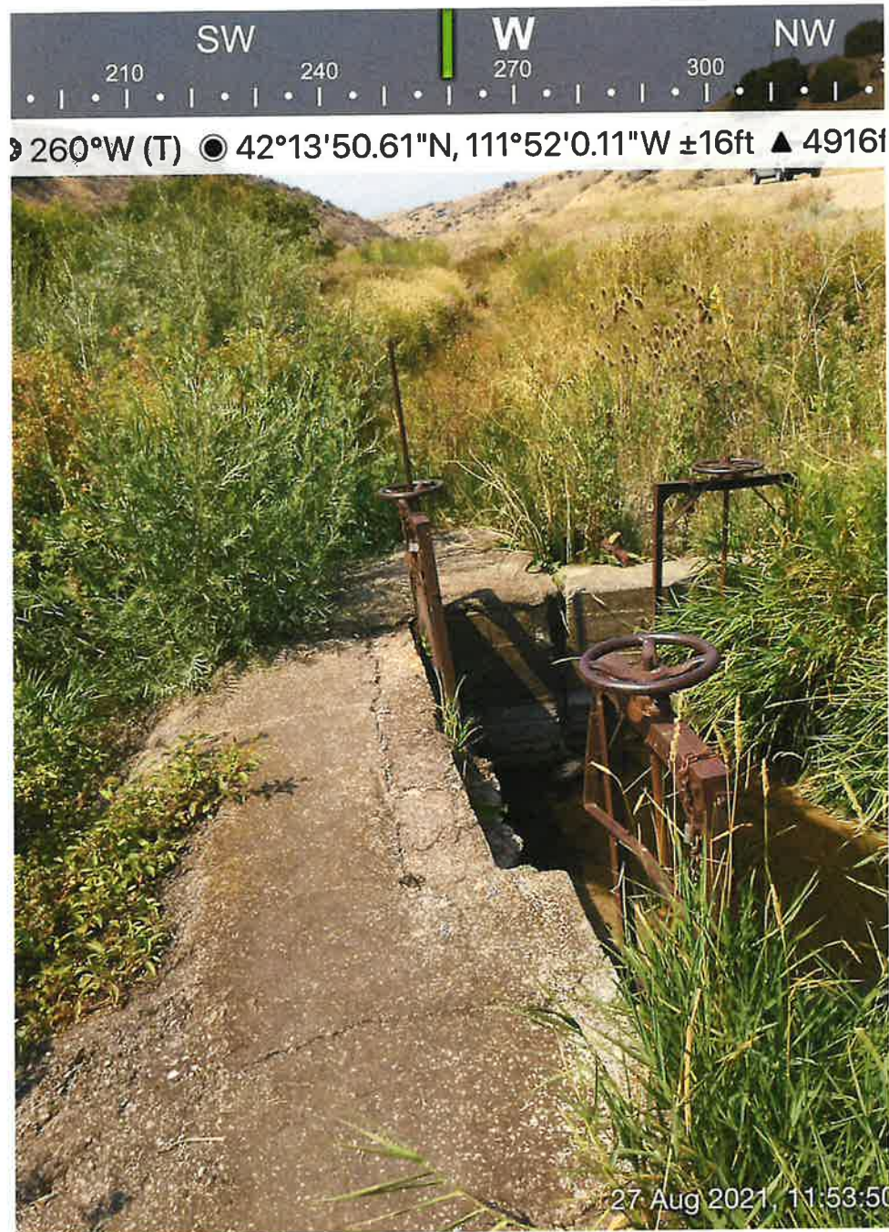
Diversion Dam and Headgate for Upper Ditch
