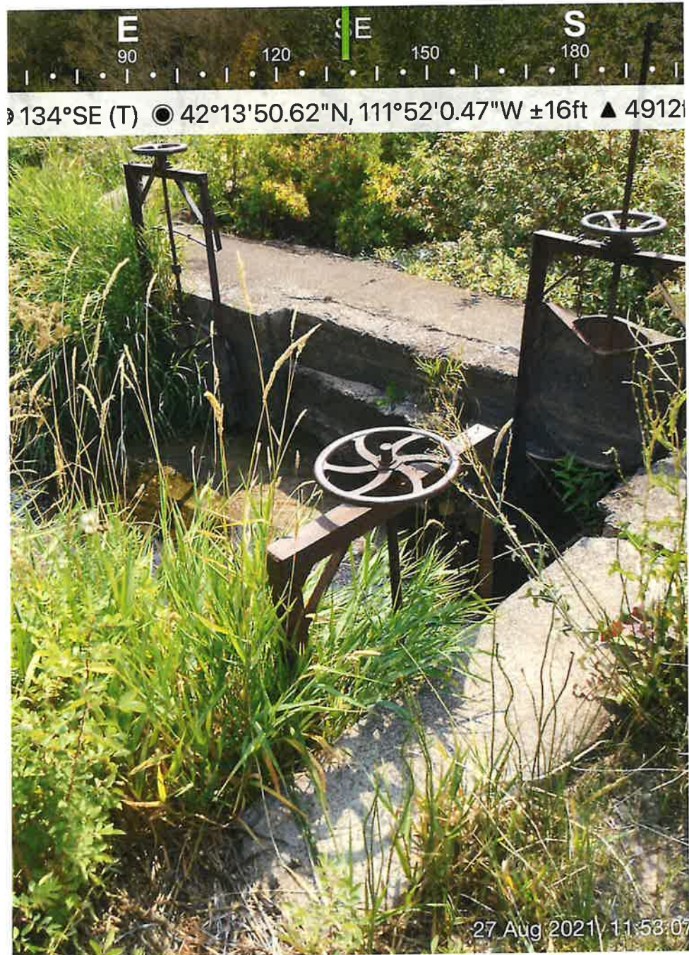
Diversion Dam and Headgate for Upper Ditch
