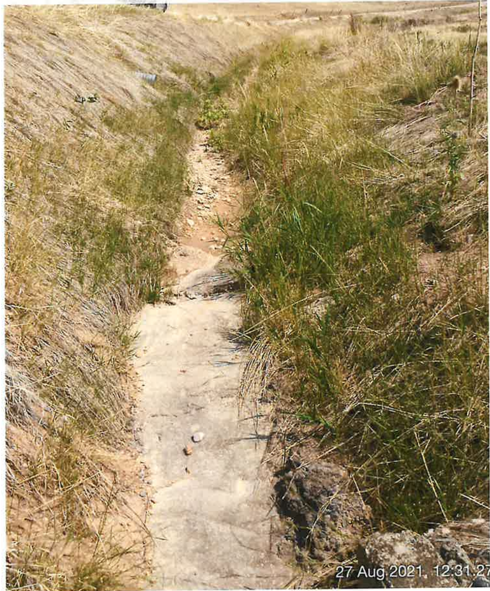
End Section of Upper Ditch
