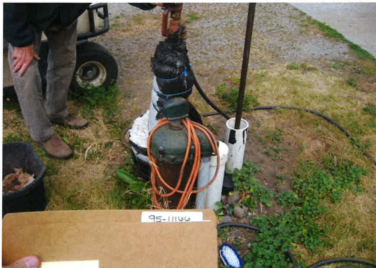
POD – OLD 1952 GROUNDWATER WELL
