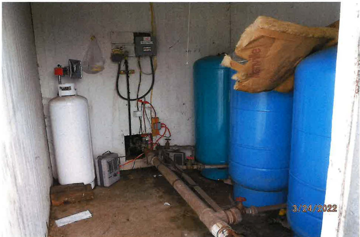
DIVERTING WORKS – 3EA PRESSURE TANKS INSTALLED IN WATER SYSTEM
