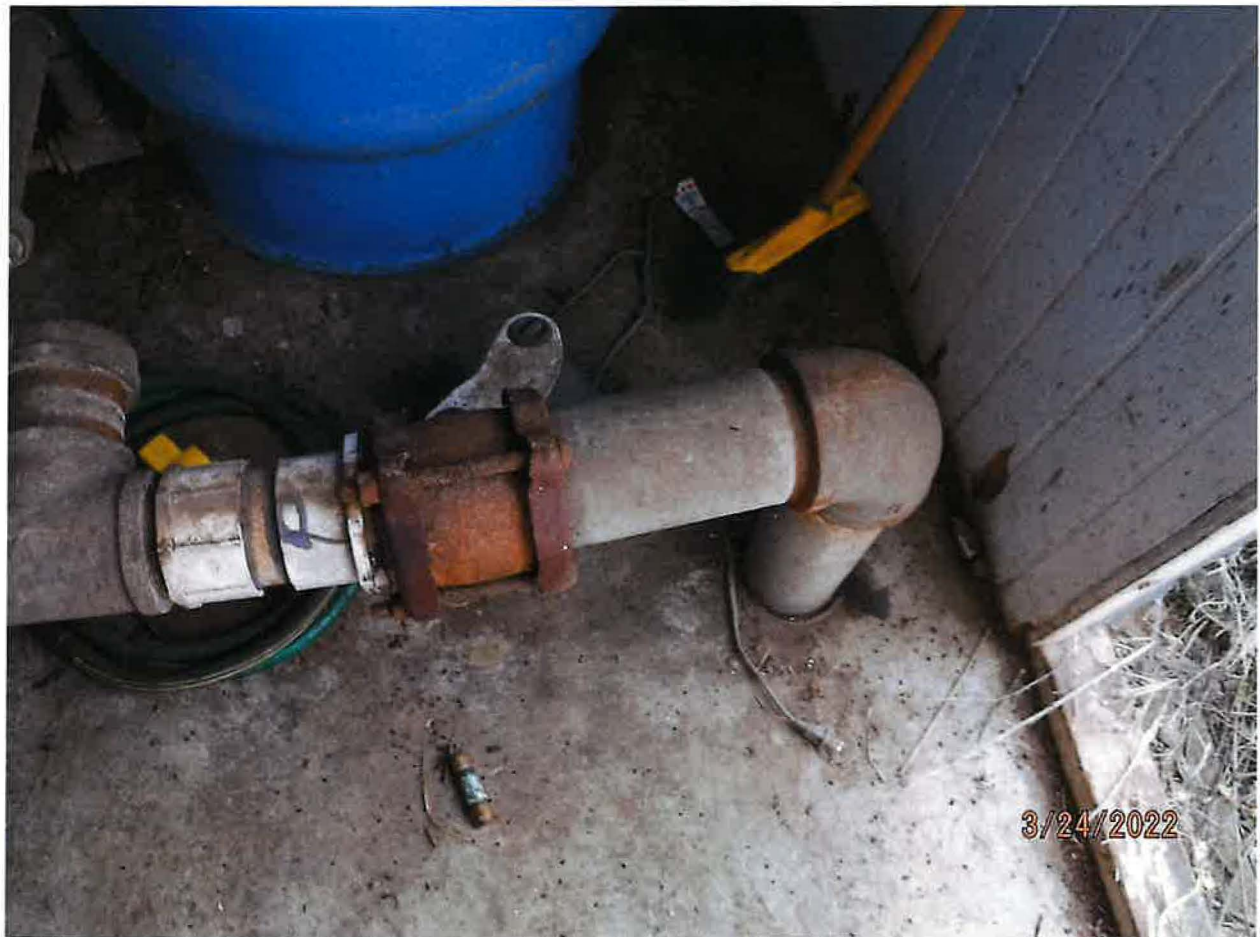
WATER SYSTEM MAIN SERVICE LINE TO POU
