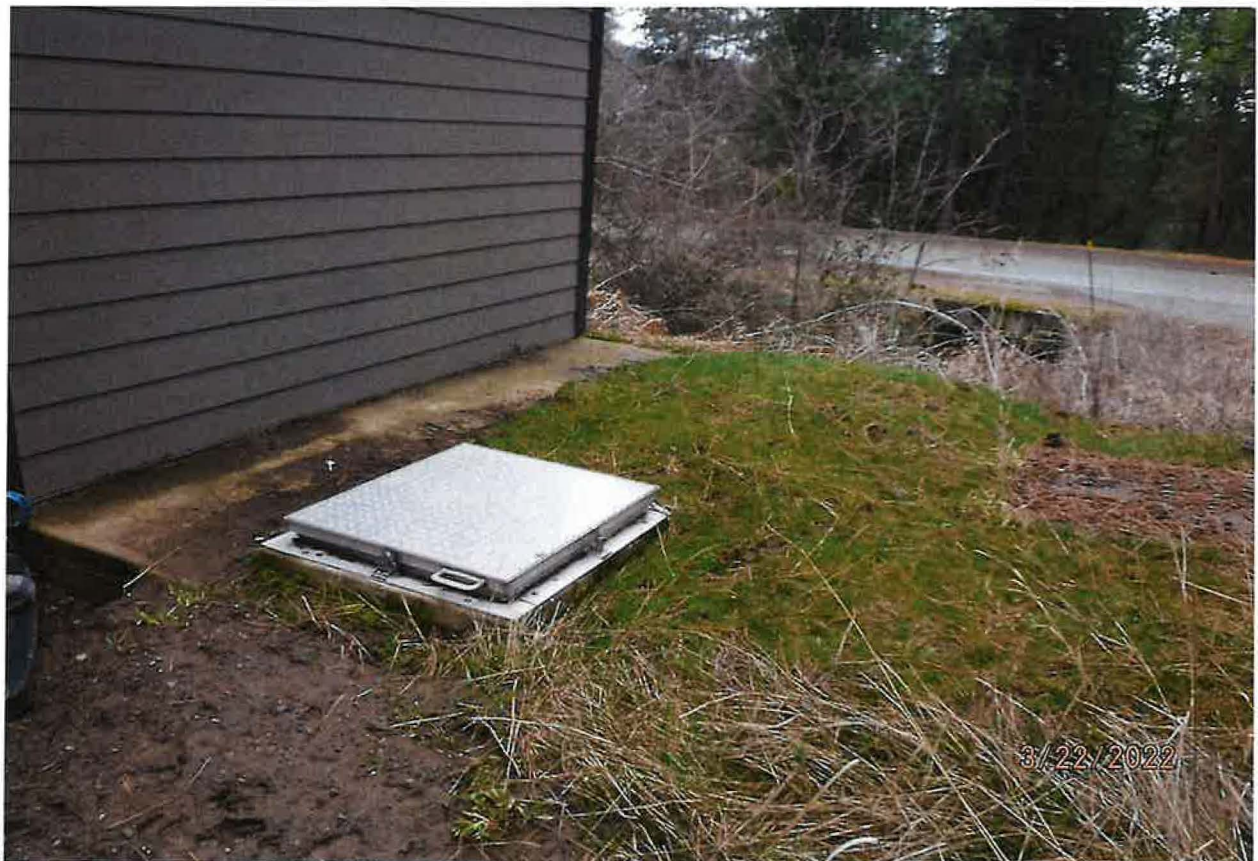
15,000 GAL STORAGE RESERVOIR
