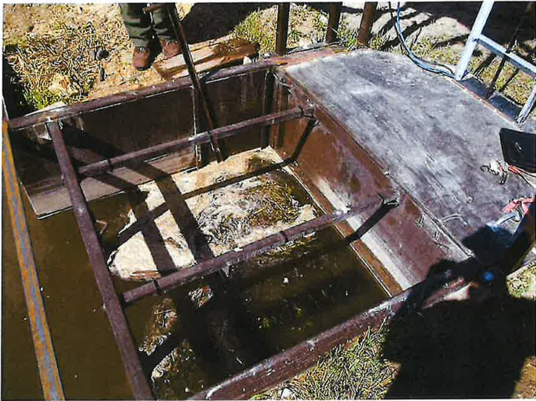
Photo 3: Close-up of fish screen structure
