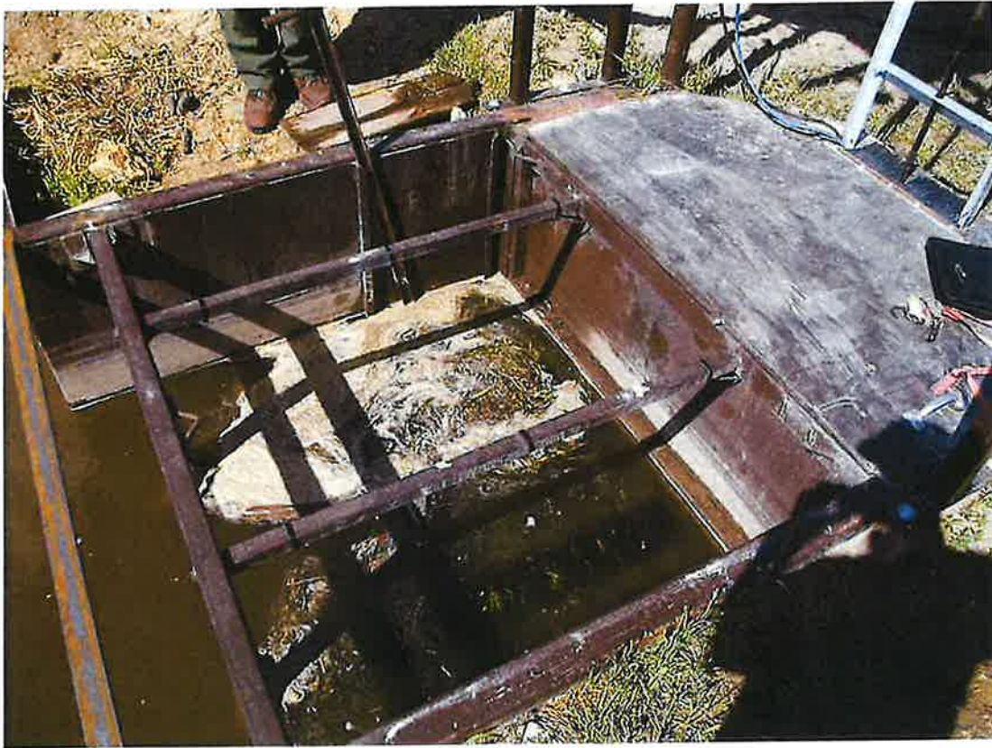
Photo 3: Close-up of fish screen structure
