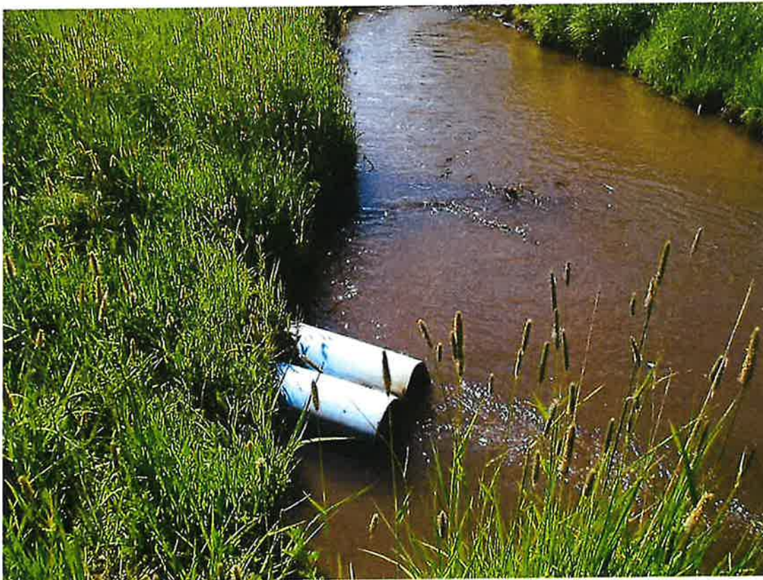
Photo 4: Fish bypass and overflow returning to Eighteen Mile Creek
