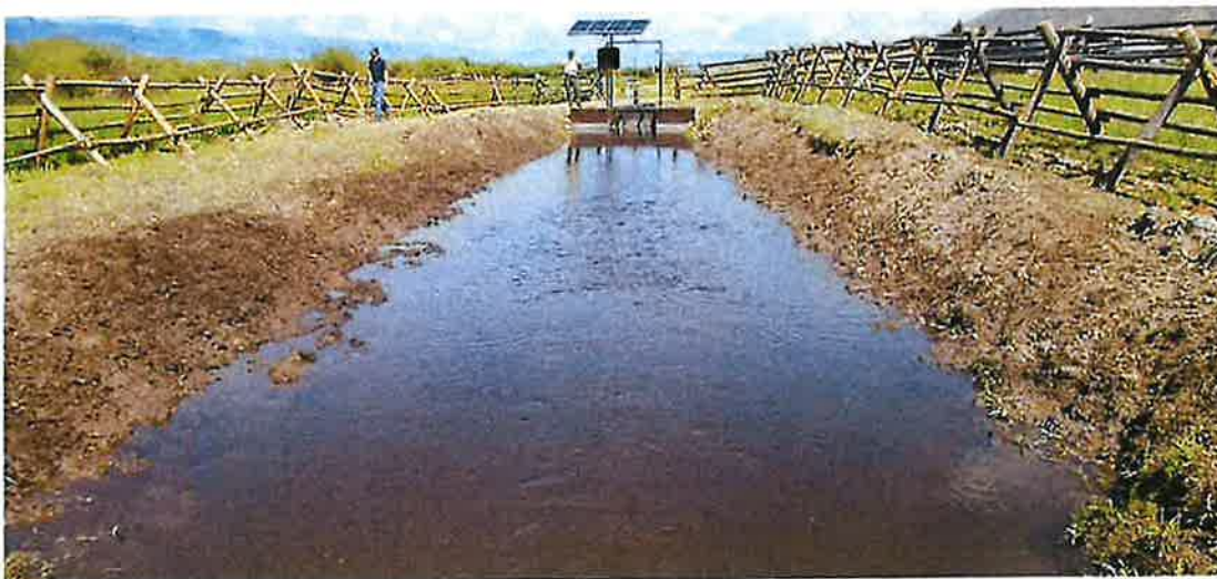
Photo 2: Fish screen/bypass approach
