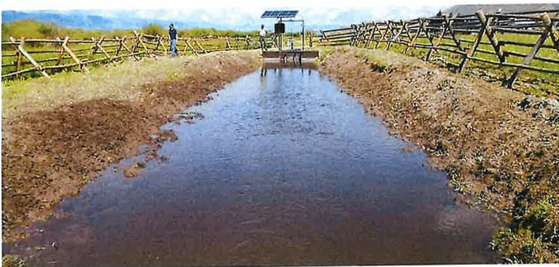
Photo 2: Fish screen/bypass approach
