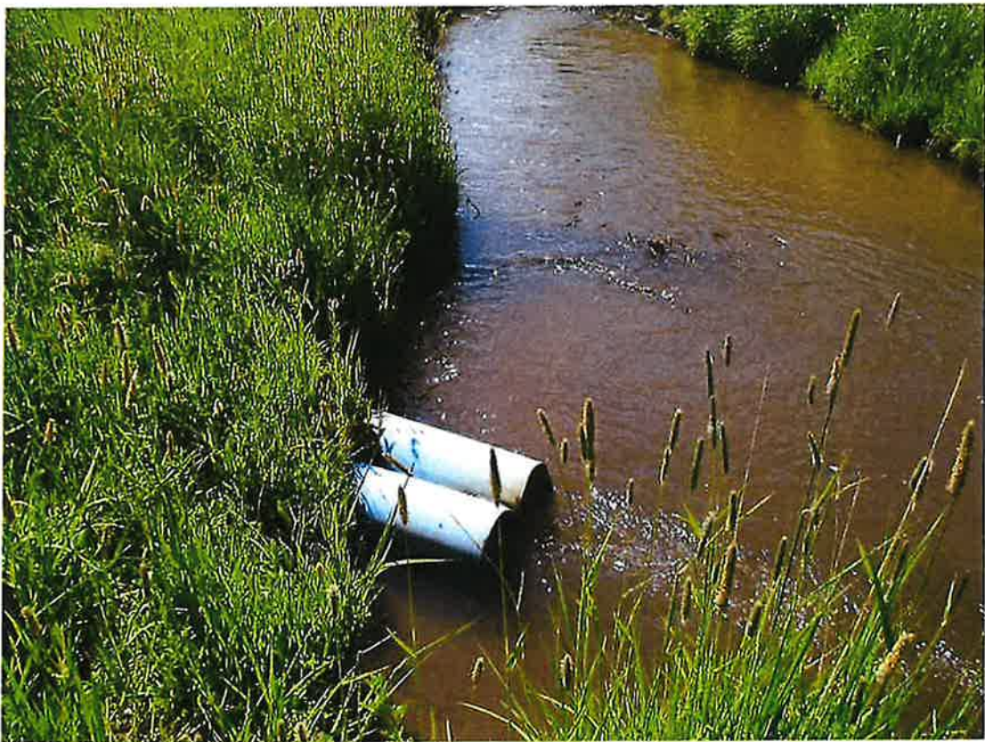
Photo 4: Fish bypass and overflow returning to Eighteen Mile Creek
