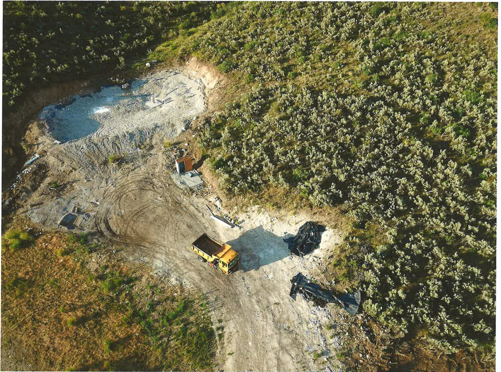
FIRE PROTECTION STORAGE POND - AS SEEN DURING CONSTRUCTION IN 2021 VIA DRONE
