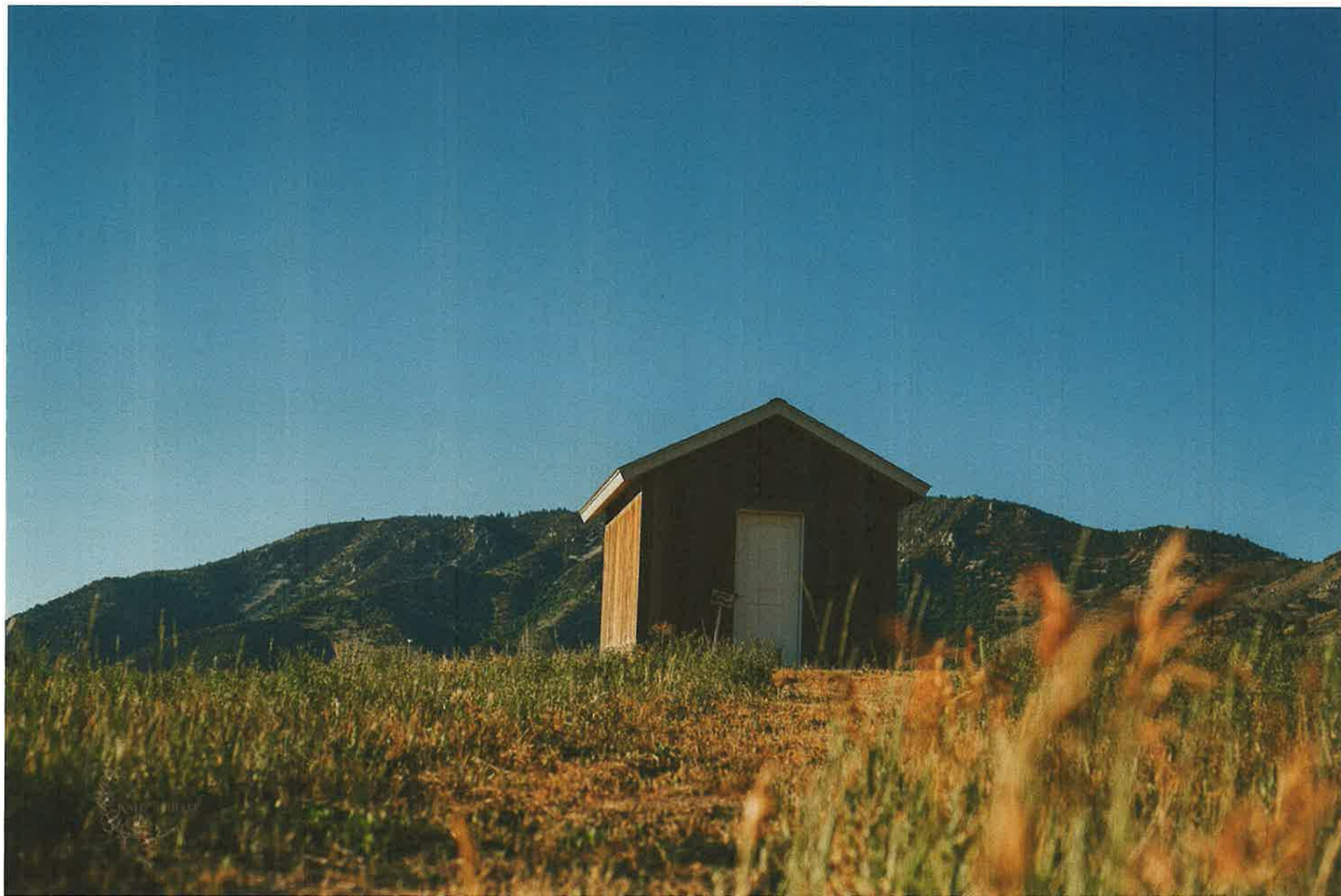
WELL HOUSE EXTERIOR AS SEEN FROM SOUTH SIDE
