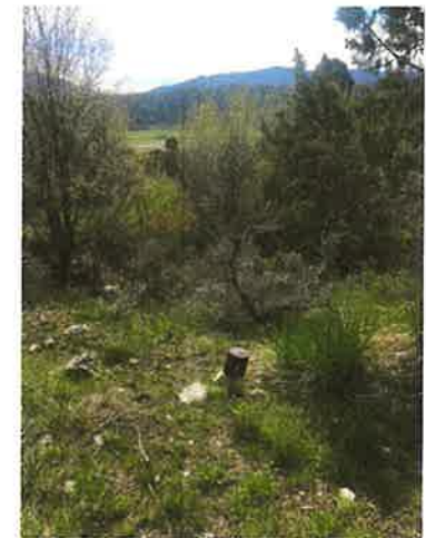
RUSTY COFFEE CAN MARKING SHUT OFF VALVE TO 500 GALLON STORAGE TANK UNDERGROUND
