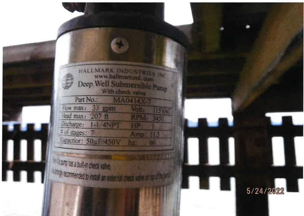
SUBMERSIBLE PUMP INSTALLED IN IRRIGATION SYSTEM
