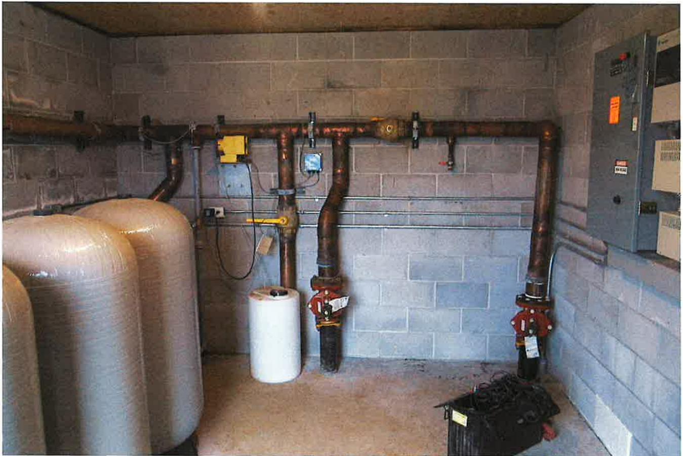
Inside well house, facing northwest.
