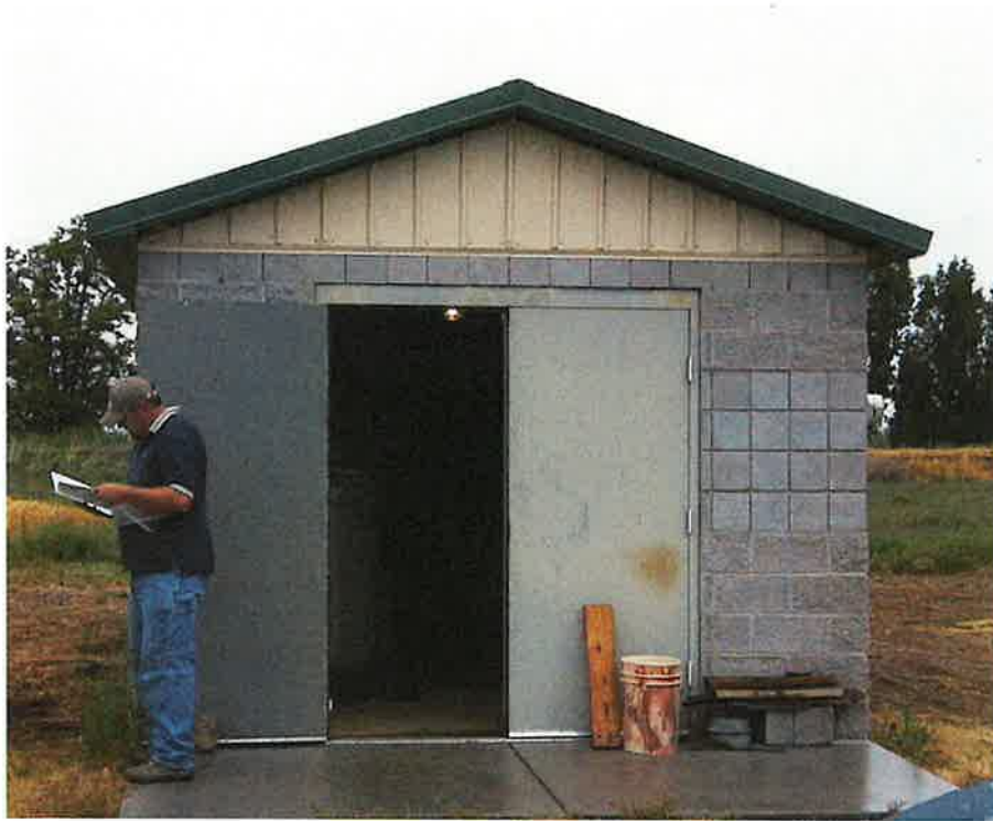
Well house, facing northwest.
