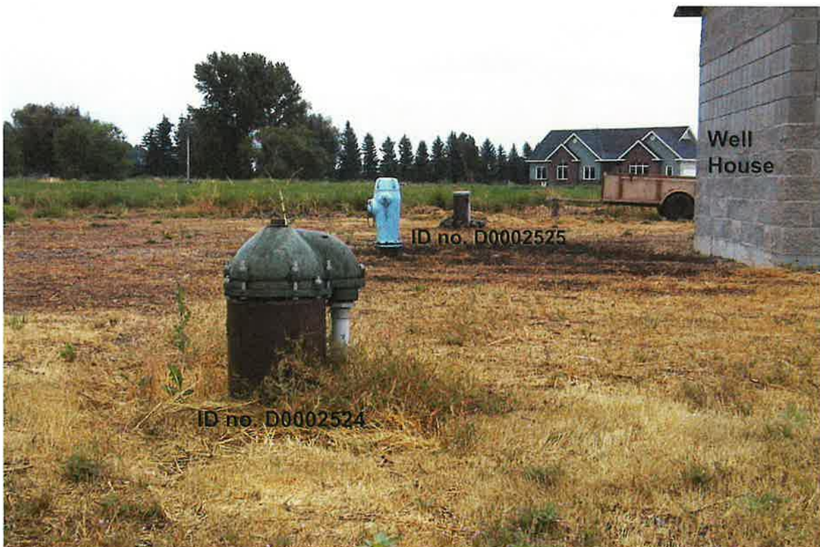
West well, in foreground with east well, in background, facing northeast.
