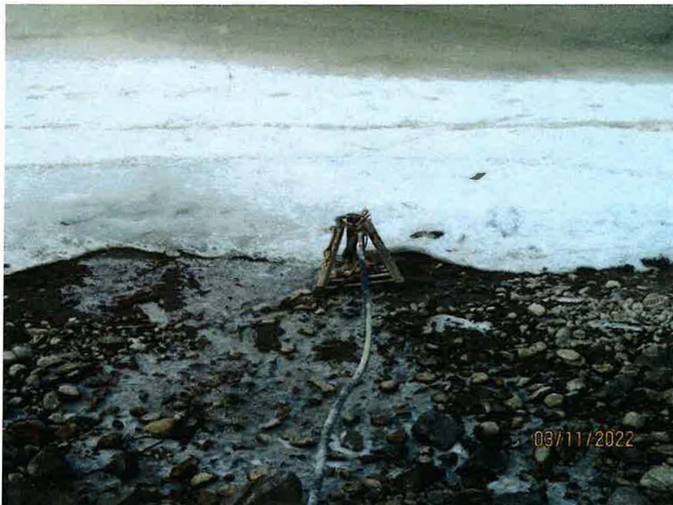
Existing SW Diversion on Parcel RP56N05W297251A in Pend Oreille River – Used for Irrigation
