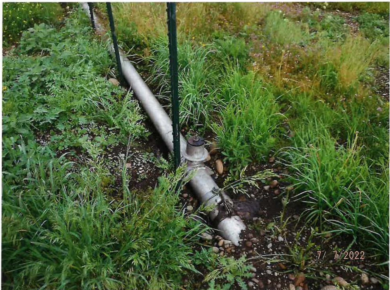
IRRIGATION POU – 8 INCH MAIN TRUNK LINE DOWN TO 4 INCH & 3 INCH HAND LINE
