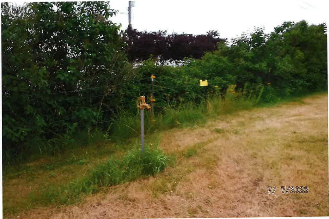
IRRIGATION POU – FROST FREE HYDRANT ALONG ROAD FRONTAGE
