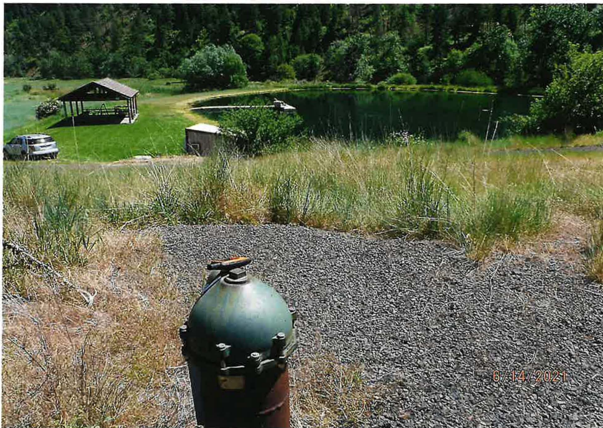
POD – GROUNDWATER WELL WITH TAG D0041142 (WELDED UPSIDE DOWN TO CASING)
