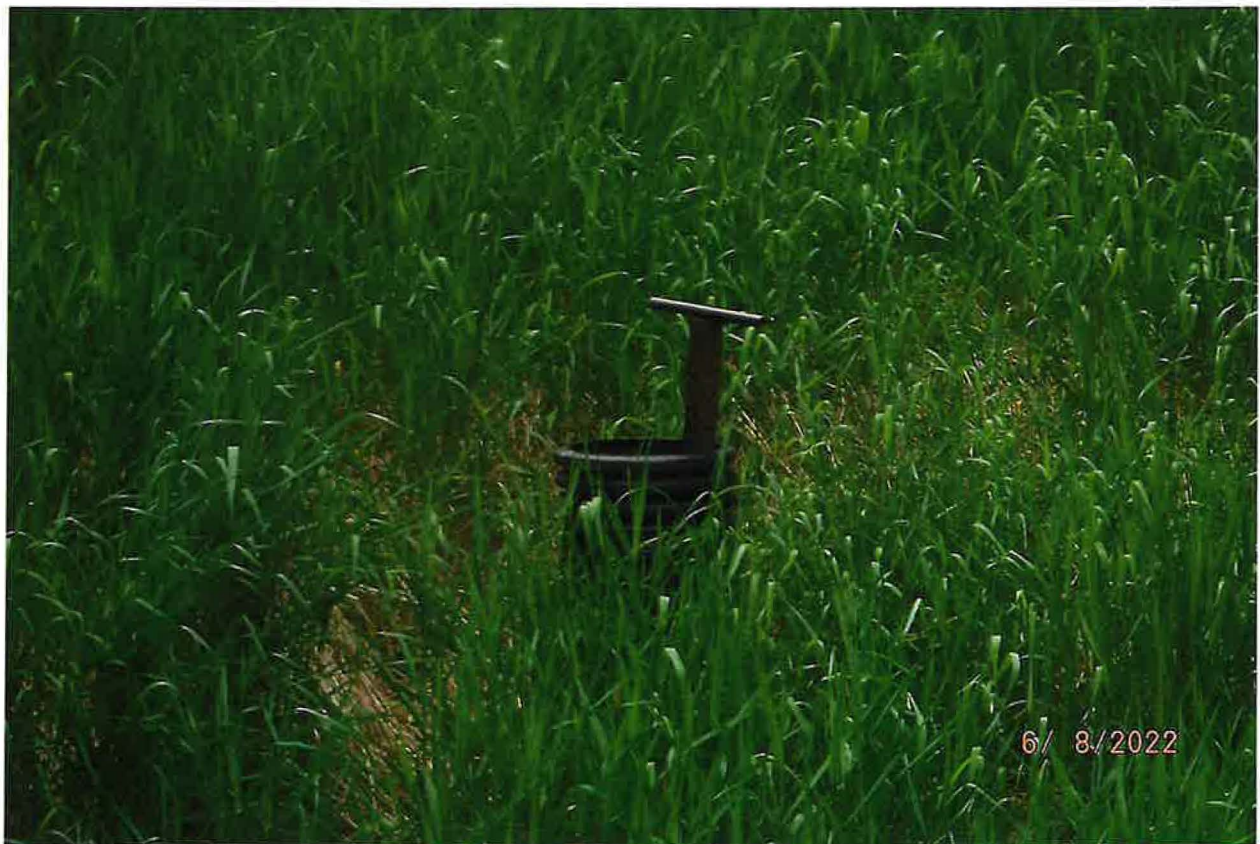
POND SET UP WITH MANUAL SHUTOFF VALVE TO FULLY DRAIN FOR MAINTENANCE
