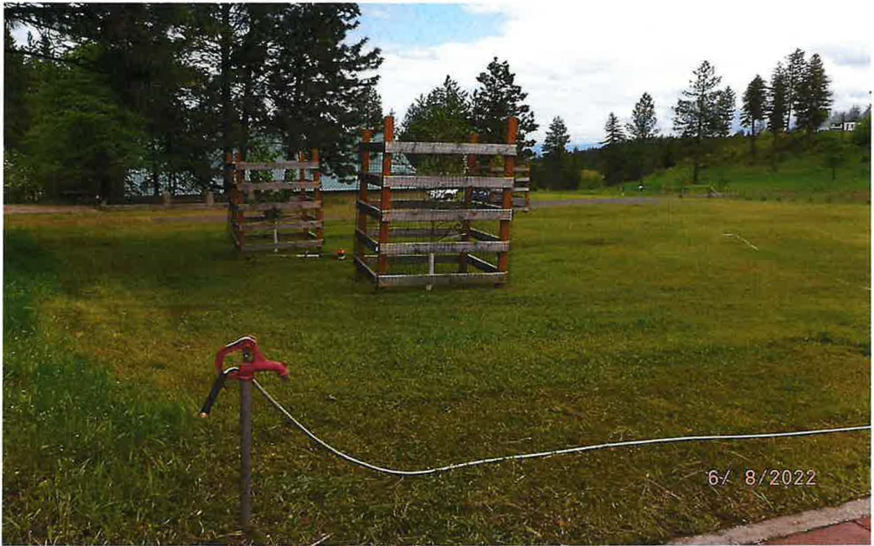
IRRIGATION FROM STORAGE POU – 2EA FROST FREE HYDRANTS RECEIVING GRAVITY FLOW FROM POND VIA BURIED POLY PIPE
