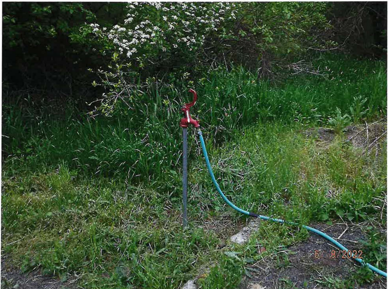
IRRIGATION FROM STORAGE POU – 2EA FROST FREE HYDRANTS RECEIVING GRAVITY FLOW FROM POND VIA BURIED POLY PIPE
