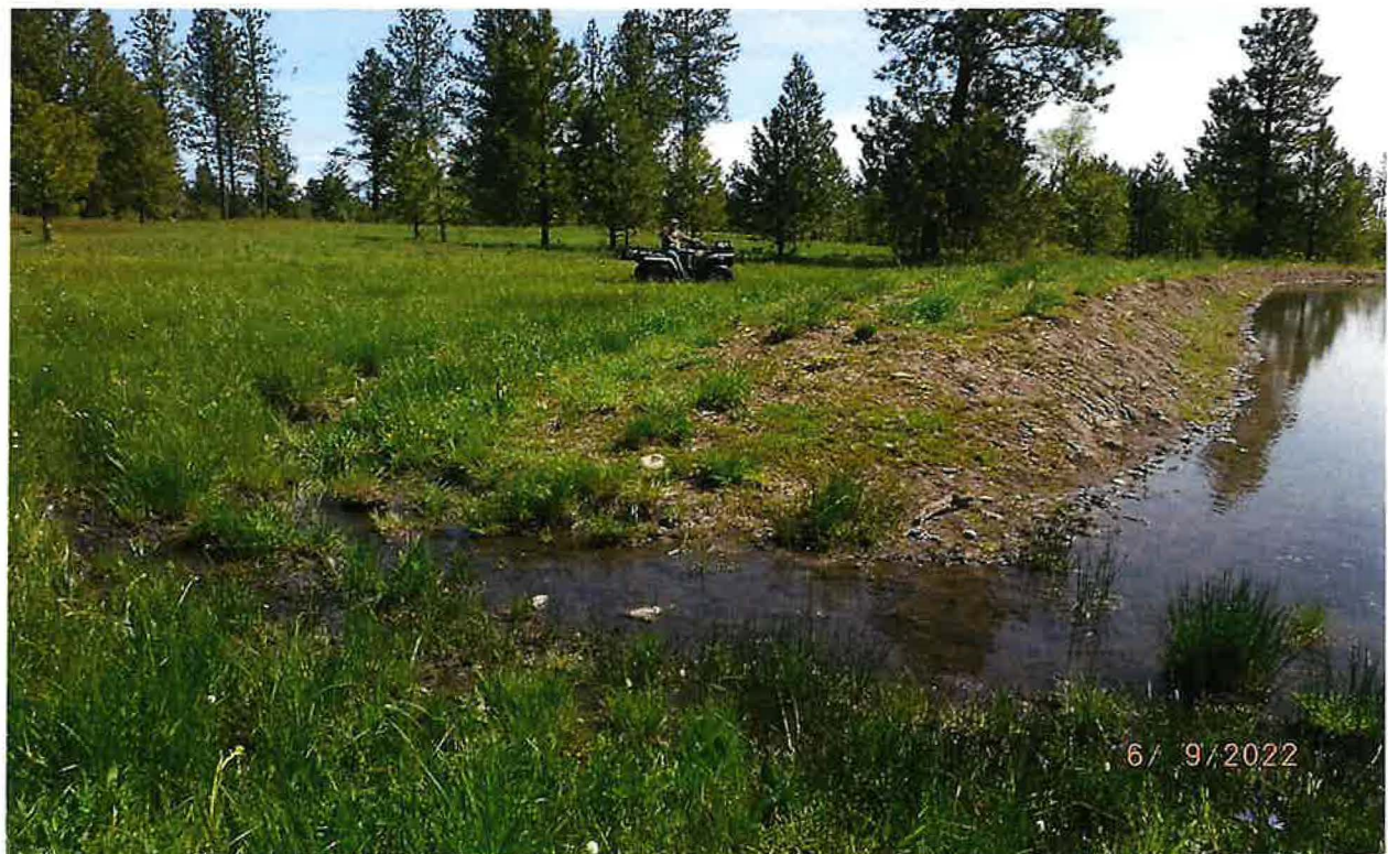
POD – EARTHEN POND DAM
