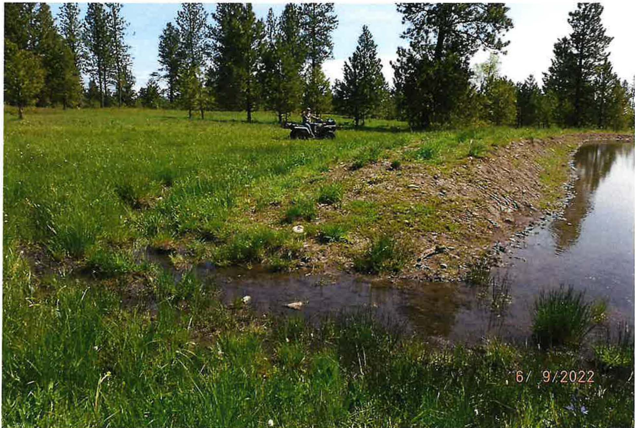
OVERFLOW DISCHARGE FROM ROCKED CHANNEL RETURNS BACK TO AN INTERMITTENT STREAM
