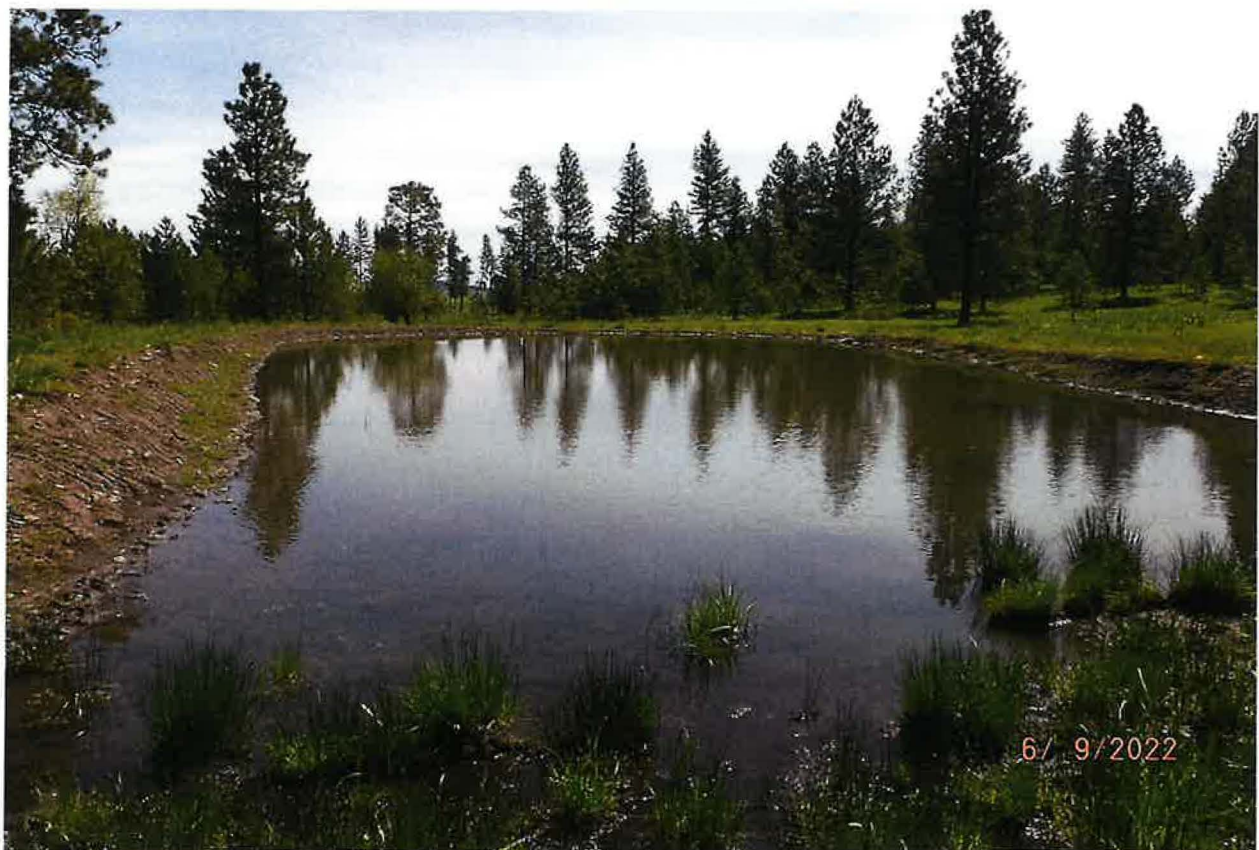
POU – STORAGE POND
