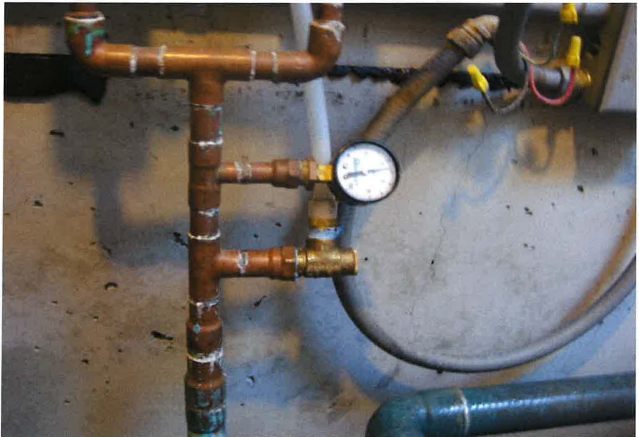
50 PSI OPERATING PRESSURE AT TIME OF EXAM
