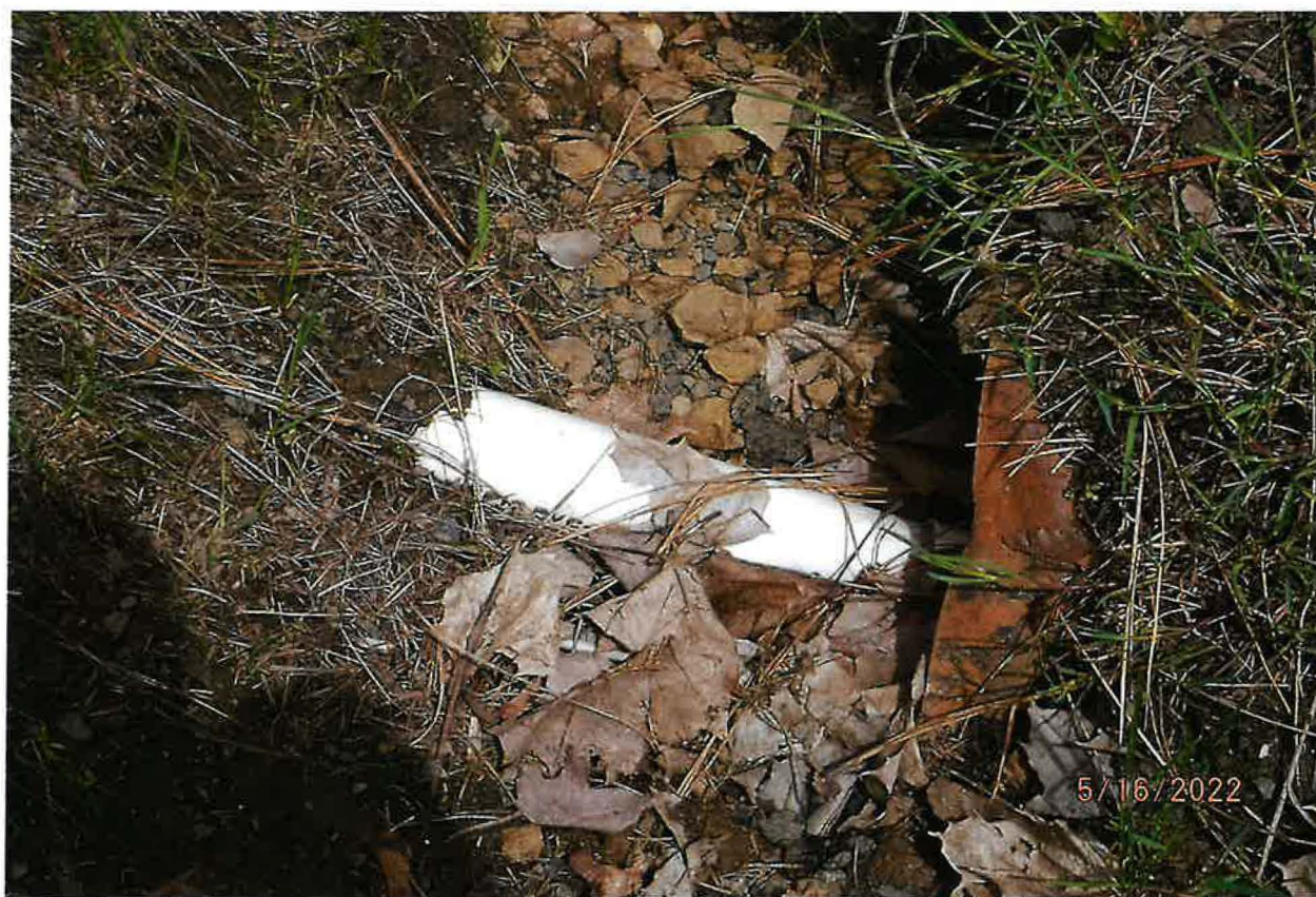
BURIED 2 INCH PVC PIPE ROUTES UPHILL APPROX 180 FT, CROSSING ROAD THROUGH A CULVERT
