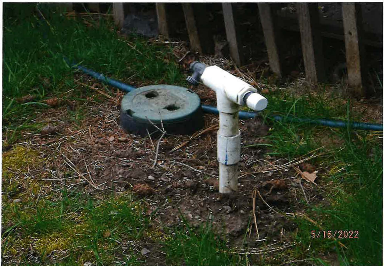
EXAMPLE IRRIGATION RISER PIPE TO HOSE BIB
