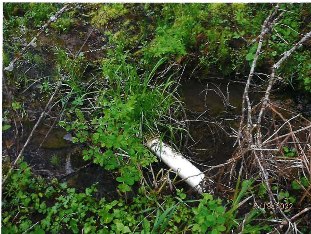
MANUAL SHUTOFF VALVE – PVC PIPE CAN BE USED TO DRAIN POND ENTIRELY FOR MAINTENANCE
