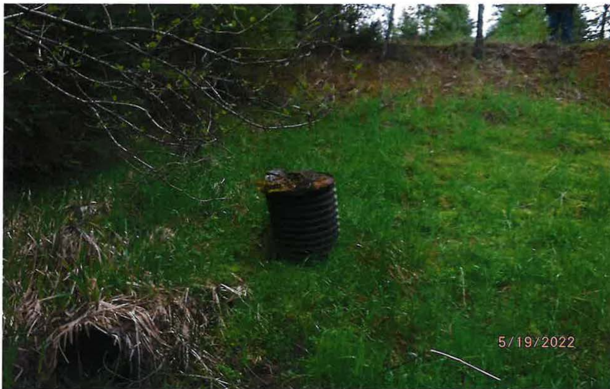
MANUAL SHUTOFF VALVE – PVC PIPE CAN BE USED TO DRAIN POND ENTIRELY FOR MAINTENANCE
