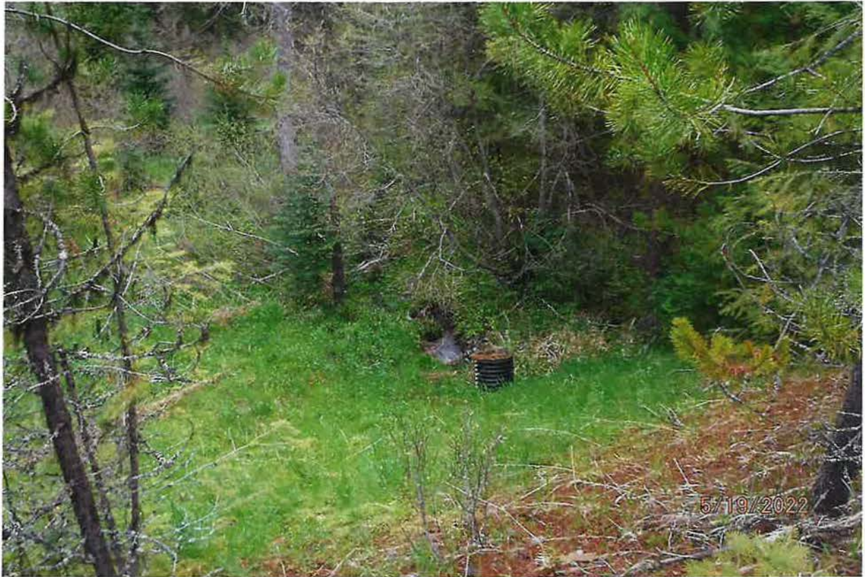
DOWNSTREAM VIEW FROM POND DAM
