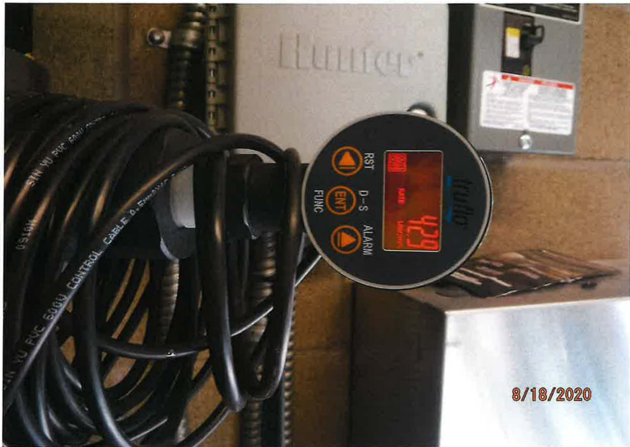
FLOW METER WELL 3 – 42.9 LITERS/MIN
