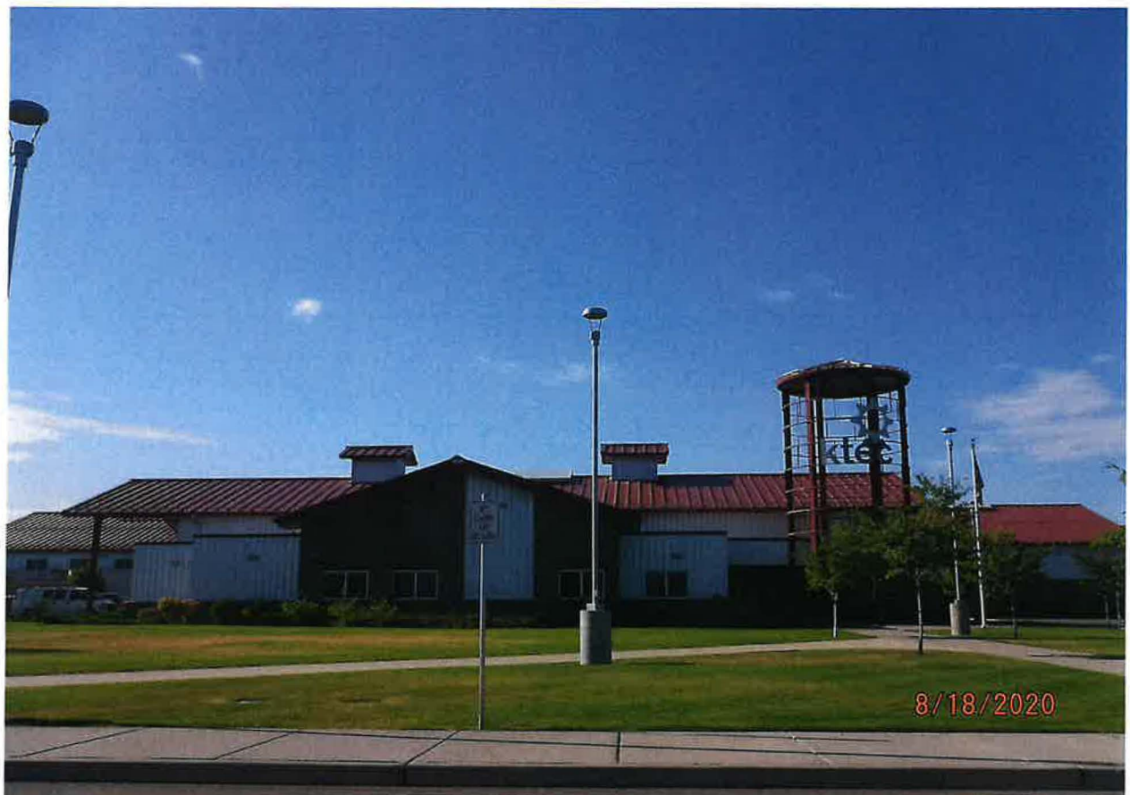
HEATING AND COOLING POU – KOOTENAI TECHNICAL EDUCATION CAMPUS
