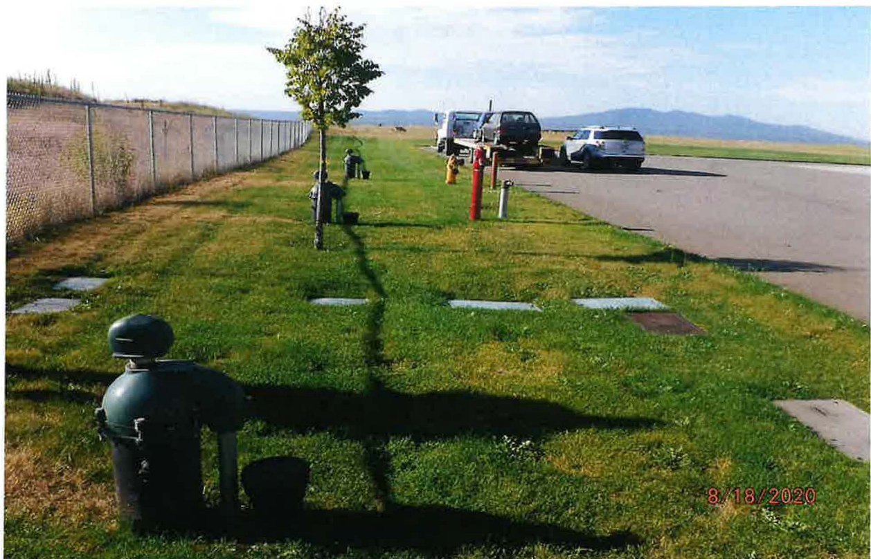
GROUNDWATER POD 3 & 4 OF 4 - FRONT AND BACK IN PHOTO – WELL D-TAG D0060949 & D0060950 (PRODUCTION WELLS)
