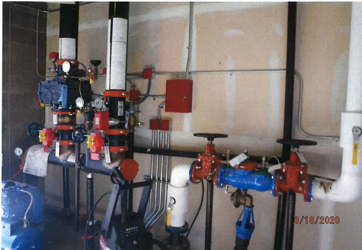
WATER CONVEYANCE SYSTEM
