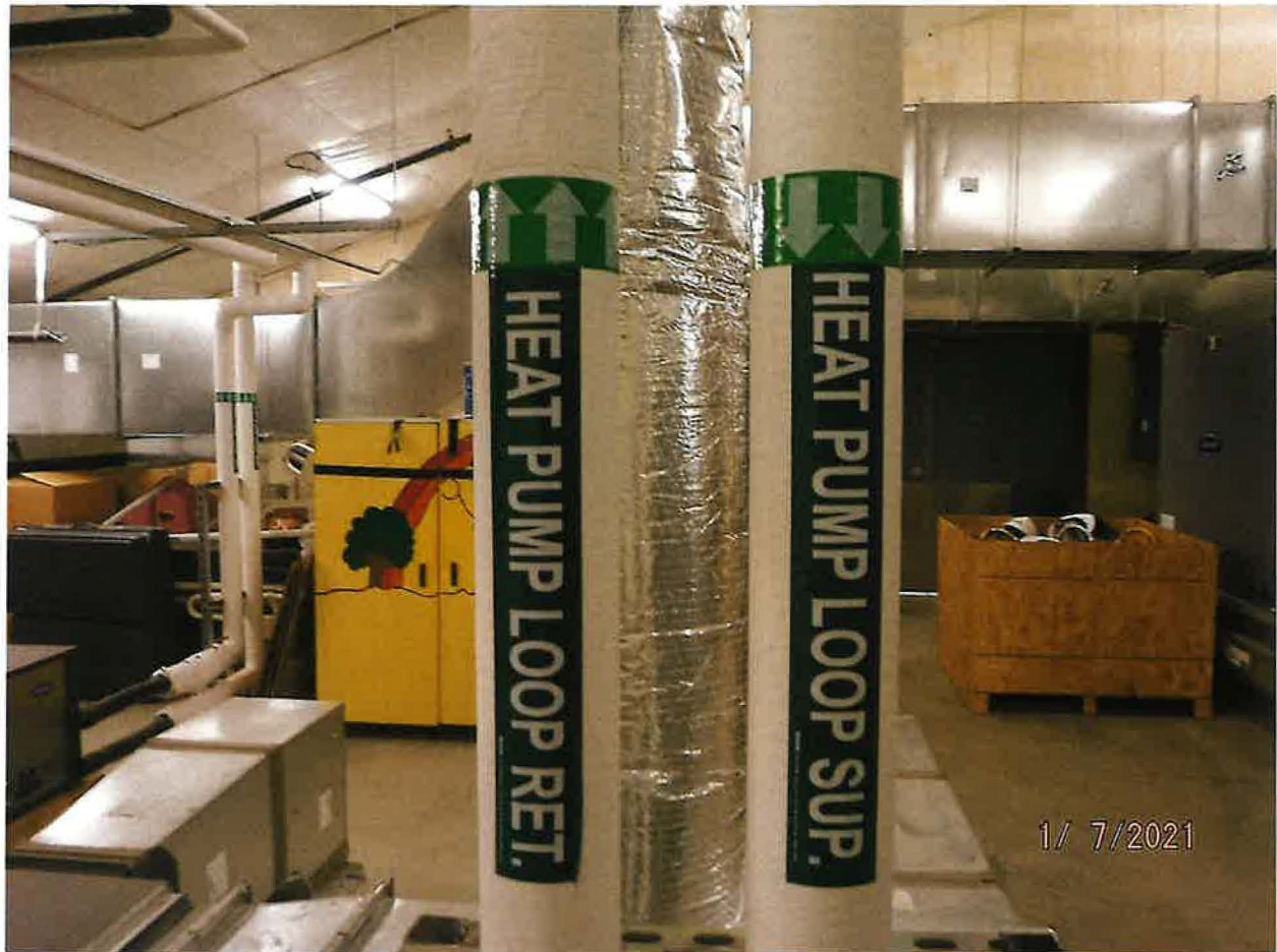
INSULATED HEAT PUMP LOOP LINE(S)
