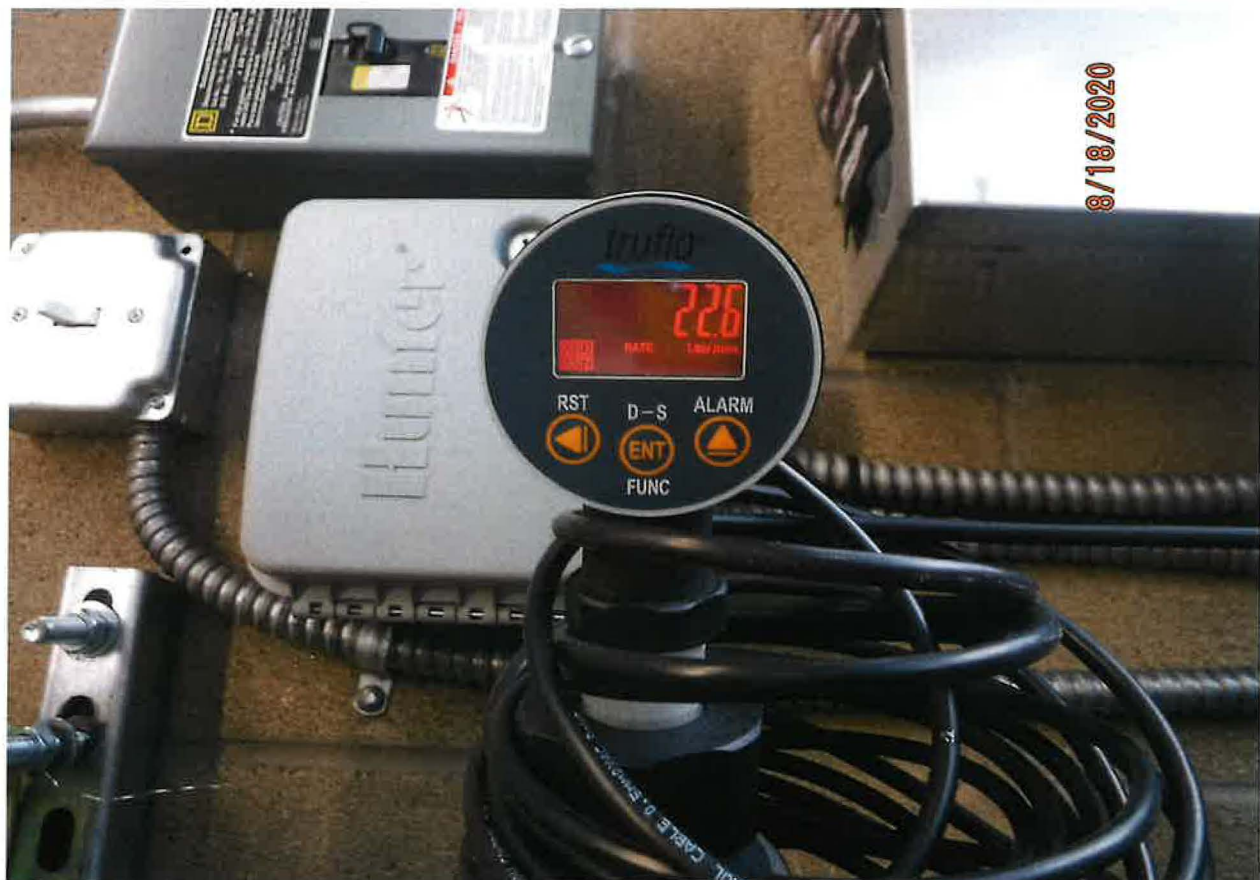
FLOW METER WELL 2 - 22.6 LITERS/MIN
