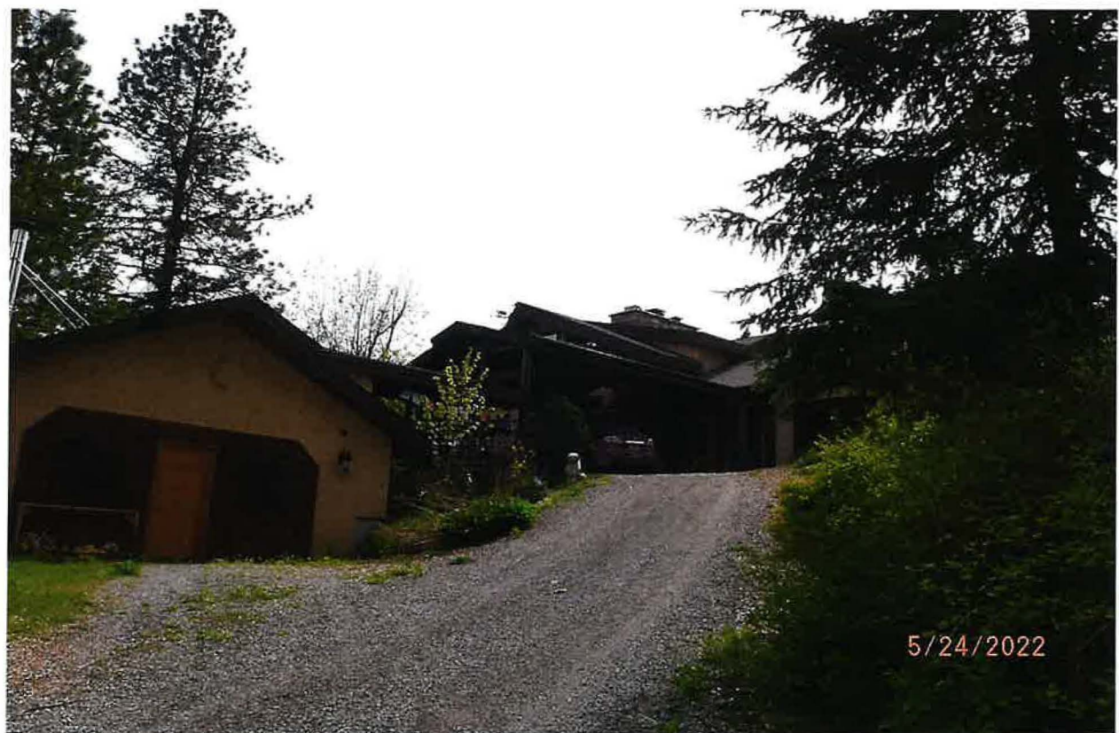
DOMESTIC POU & COMMERCIAL POU – RESIDENCE IN BACKGROUND OF PHOTO, SHOP CONVERTED INTO COMMERCIAL USE FACILITY FOR GROUP ACTIVITIES
