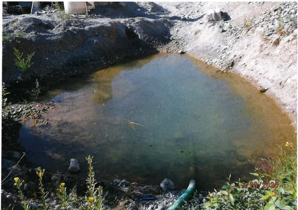
GROUND WATER SOURCE – MANMADE OPEN PIT WELL
