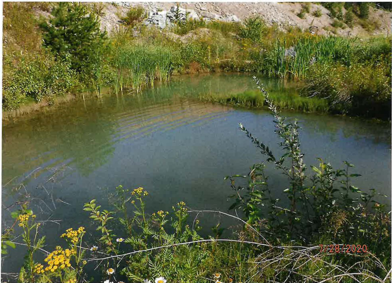
SMALL SETTLING POND FOR SILT FALL OUT BEFORE ENTERING STORAGE POU
