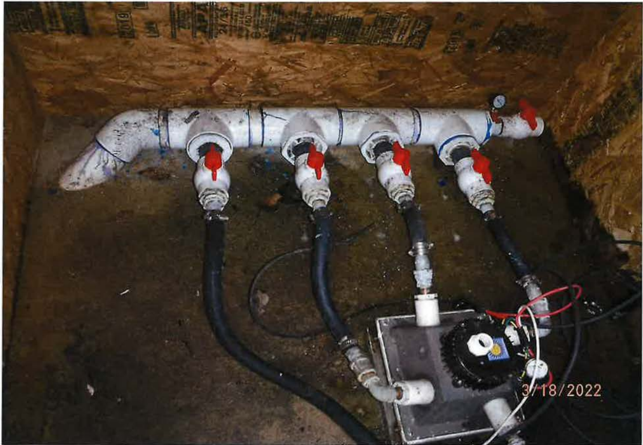
POWER POU – HIPOWER HYDROELECTRIC TURBINE LV1500; 1EA 3/16 INCH NOZZLE & 3 EA 1/4 INCH NOZZLES
