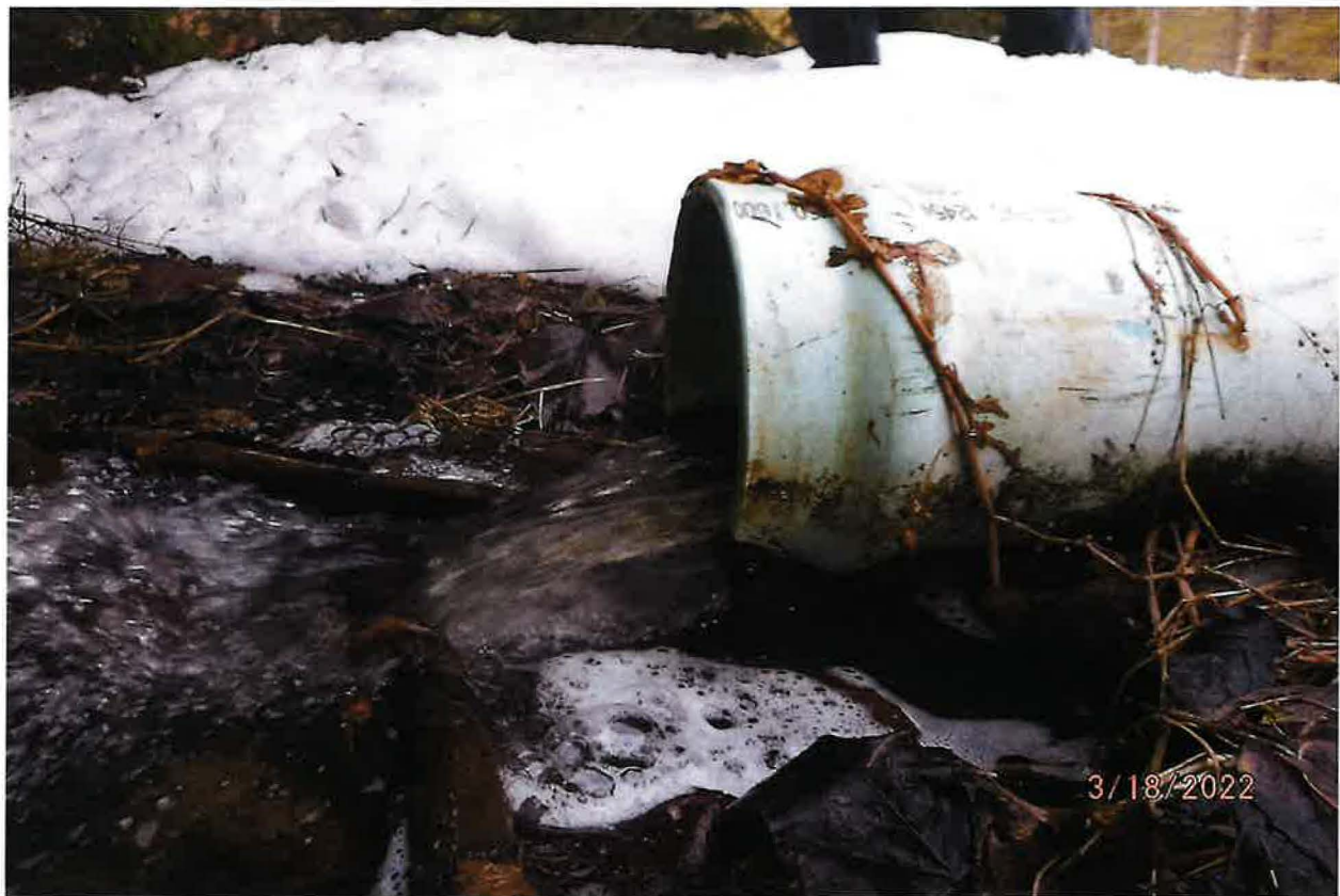
OVERFLOW DISCHARGE WITH 4EA HEADS GENERATING POWER
