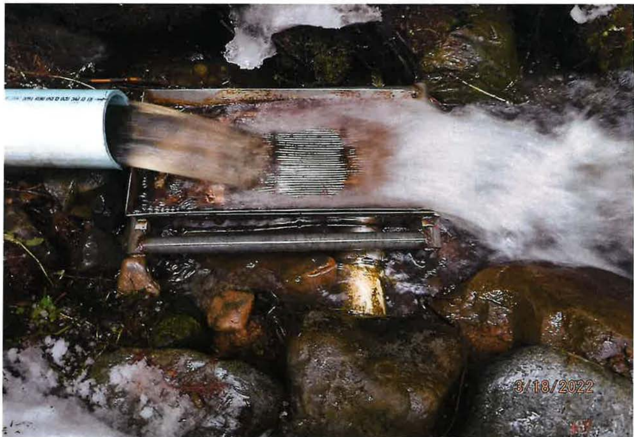
AT POD – SCREENED INFLOW TO PENSTOCK – 4 INCH PVC PIPE IN STREAM
