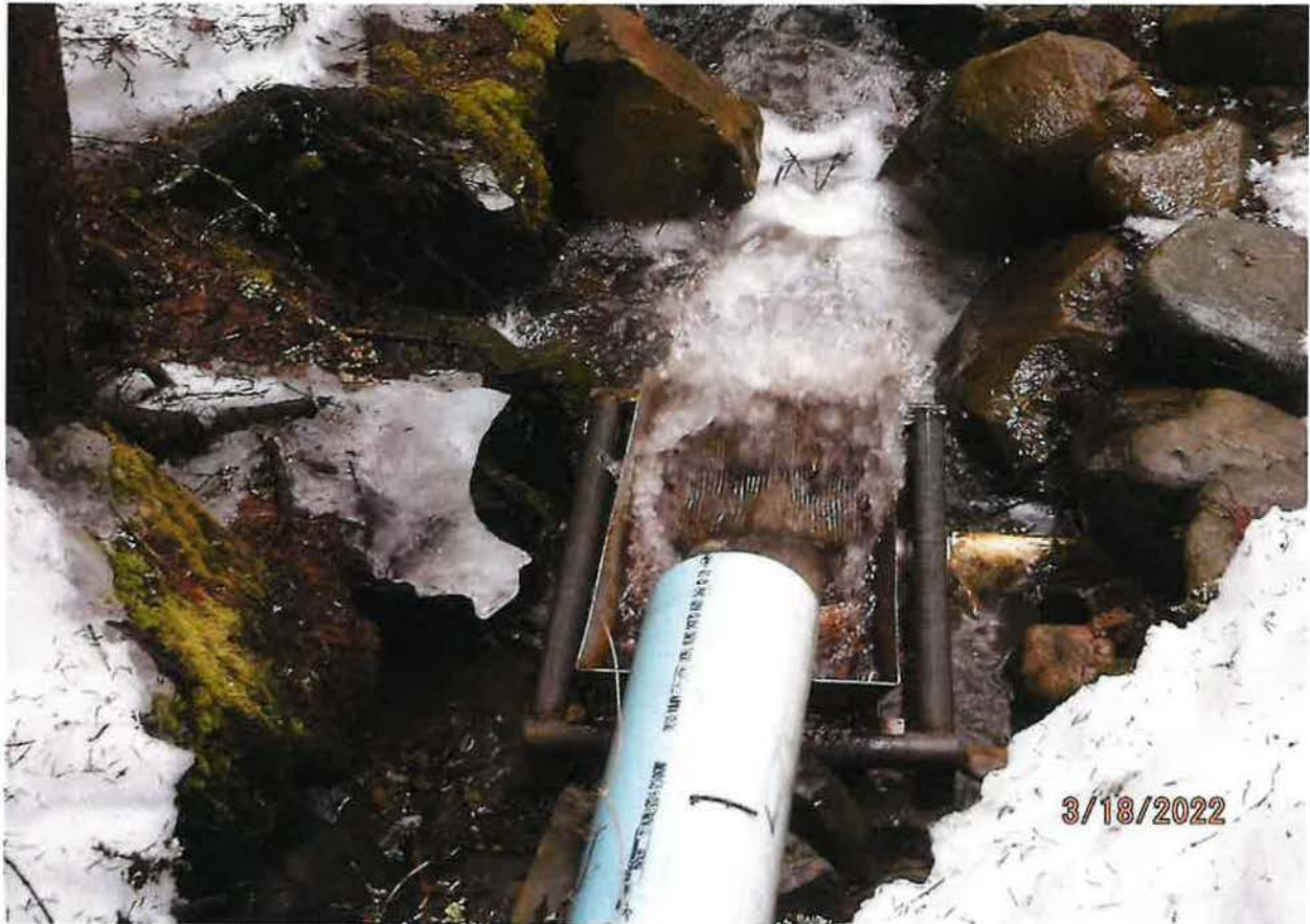
AT POD – SCREENED INFLOW TO PENSTOCK – 4 INCH PVC PIPE IN STREAM
