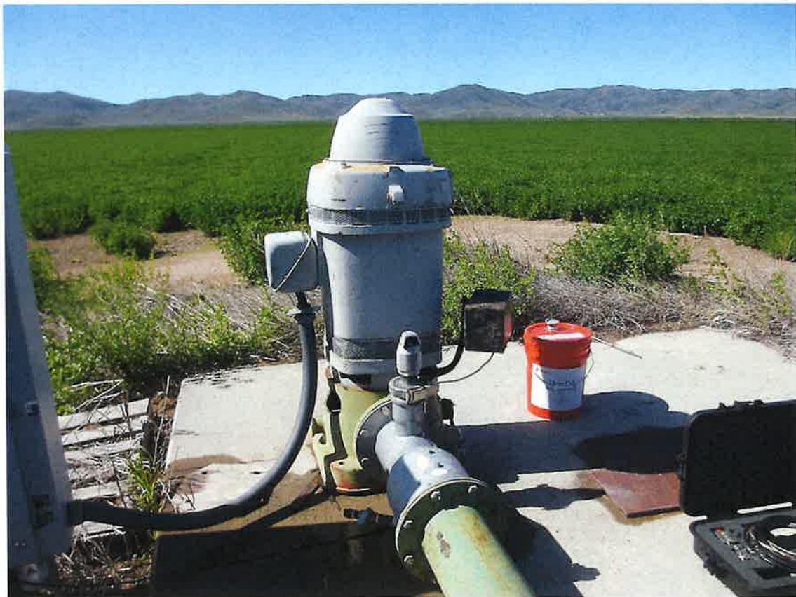
37-8057 Strom Ranches, Inc.
