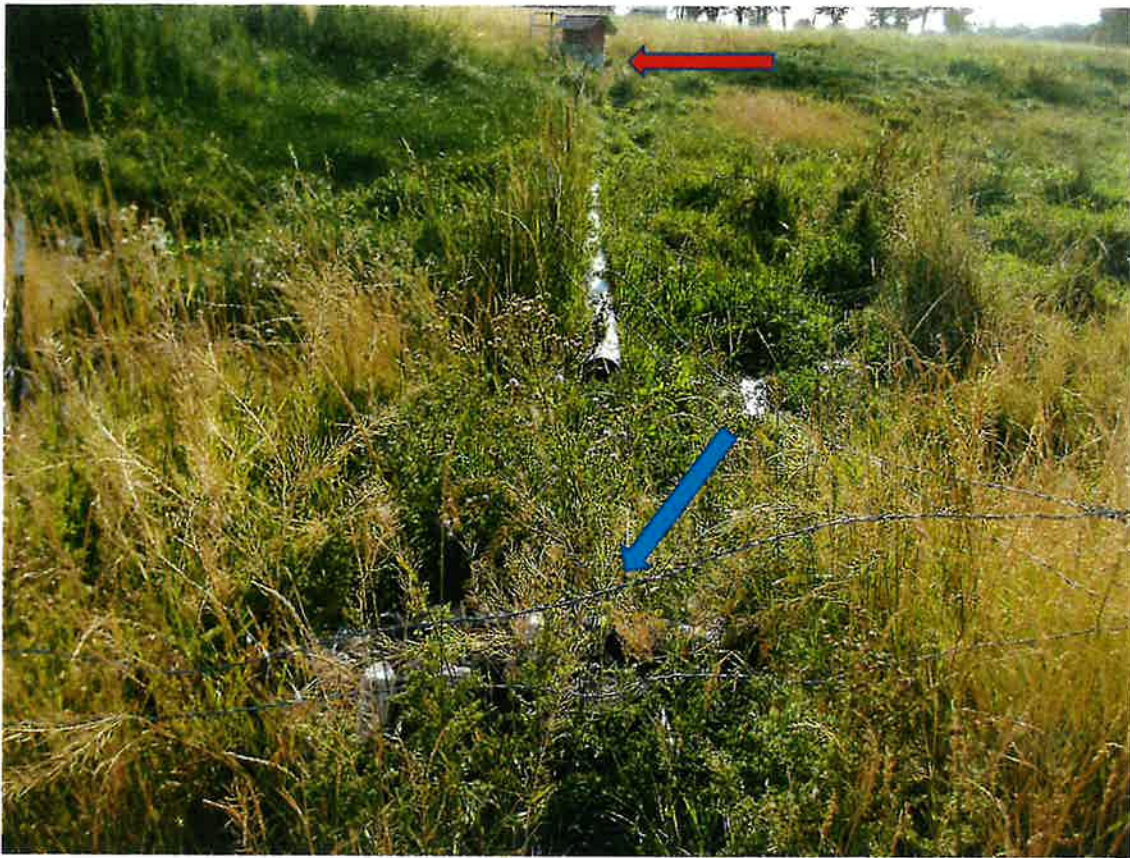
Point of Diversion (blue arrow) – Standpipe (red arrow) with booster pump in background
