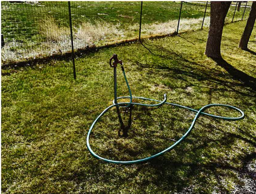
Photo 19. Kulicke hose bib on south side of yard.
