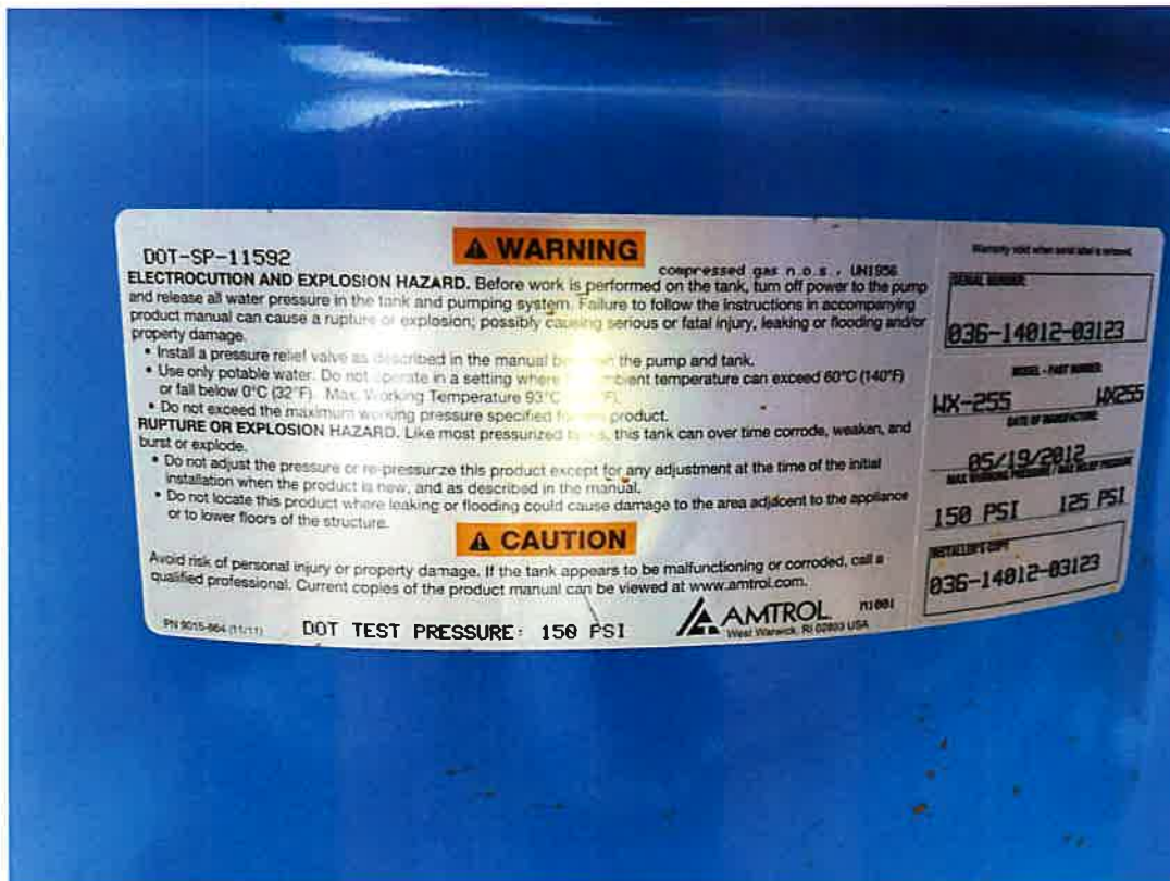
Photo 5. Hydropneumatic tank technical label, typical of each of five tanks.
