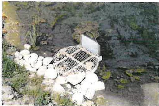
Slide gate in pond.
