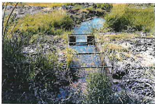
Weir below pond.
