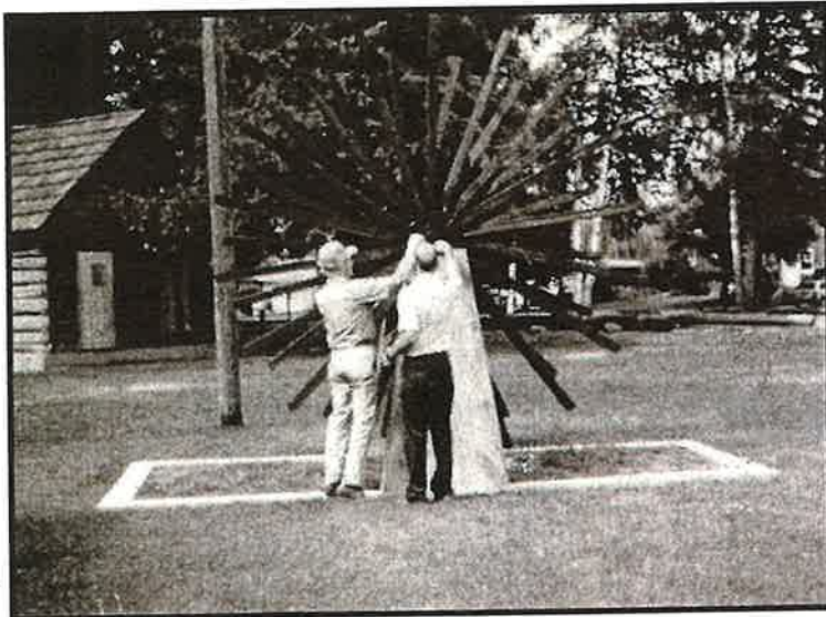
The water wheel being reconstructed in Lakeview Park; Ken Reed and Bob Kalb working on bolting the axle.
