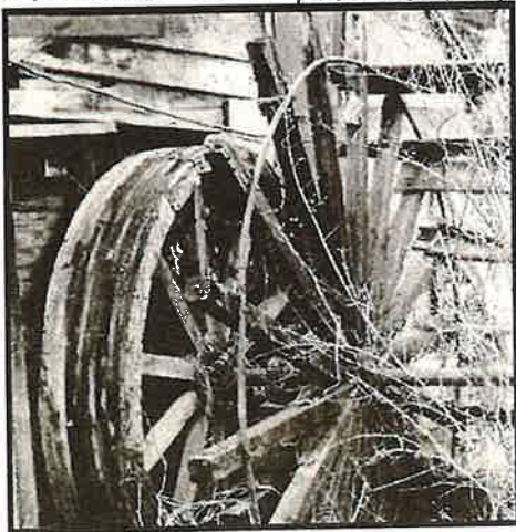
This picture shows how the water wheel looked just before being raised and removed from its place beside Hoodoo Creek.
