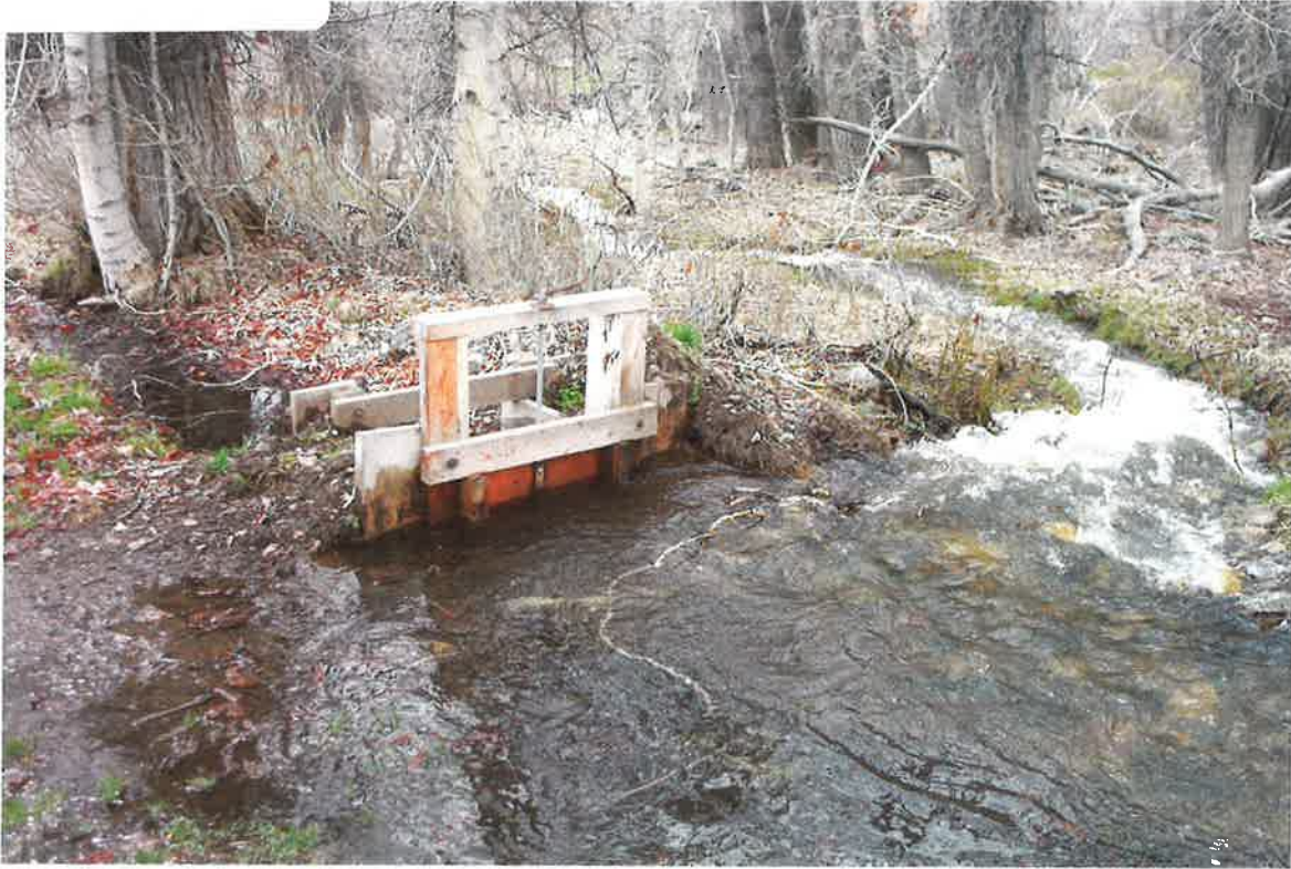
Water Right #37-12392 Head gate and Weir Argosy Creek May 9, 2005
