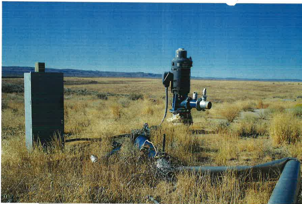
Well & Disconnected Mainline, 37-7745A Looking Easterly By J E Stanton 9-23-03
