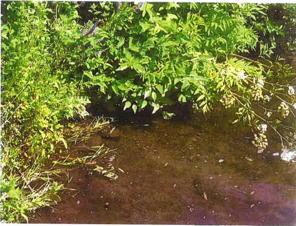
Pond end of 18" CMP.
