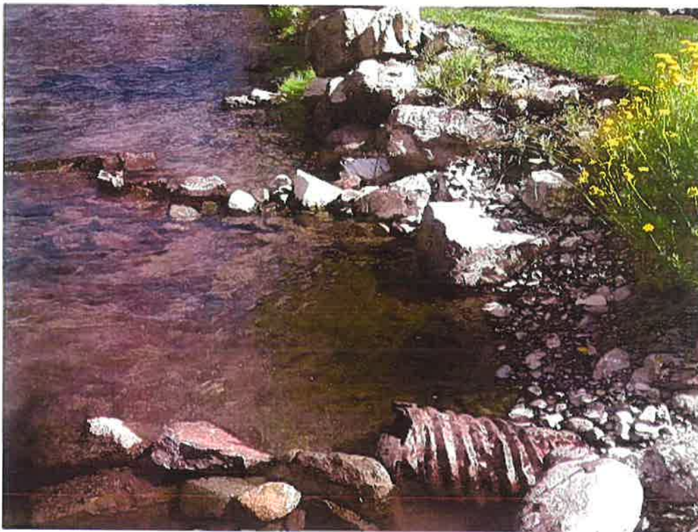
Point of diversion area: 18" CMP pipe in background, 12" CMP in foreground.
