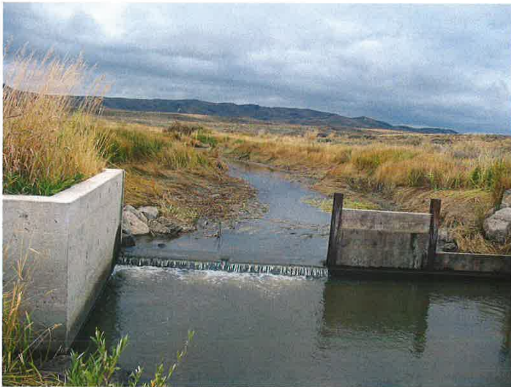
Photo of control structure for Camas Creek near POD in SWNW Sec. 5 on Camas Creek
