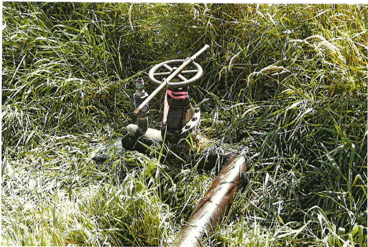
Outlet for Dreyers artesian well located in the SWSWSE of S13, T01S, R18E measured at 0.29 cfs.
