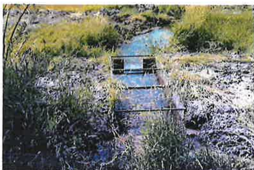
Weir below pond.
