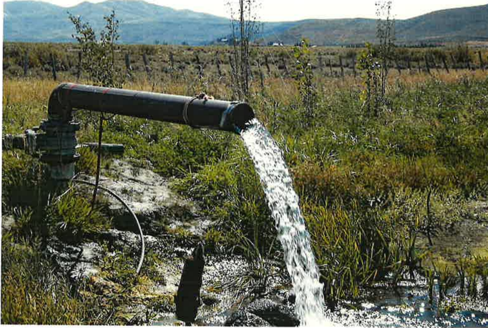
Artesian well located in the NENENE of S13, T01S, R18E. Source for Smith/Dreyer/Stasz rights/claims. Measured at 0.78 cfs with the Fuji flowmeter.
