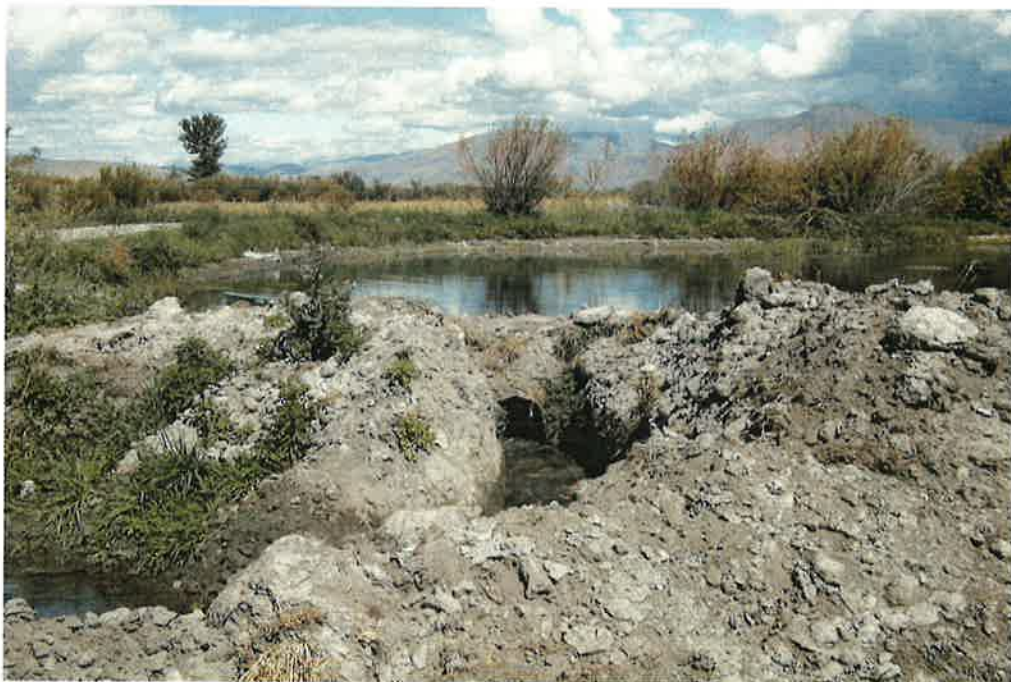
Bottom end of Smiths headgate, newly constructed culvert and ditch.
