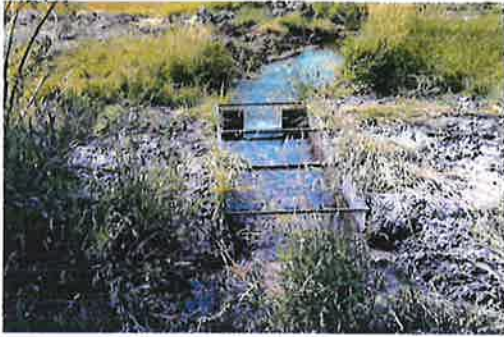
Weir below pond.
