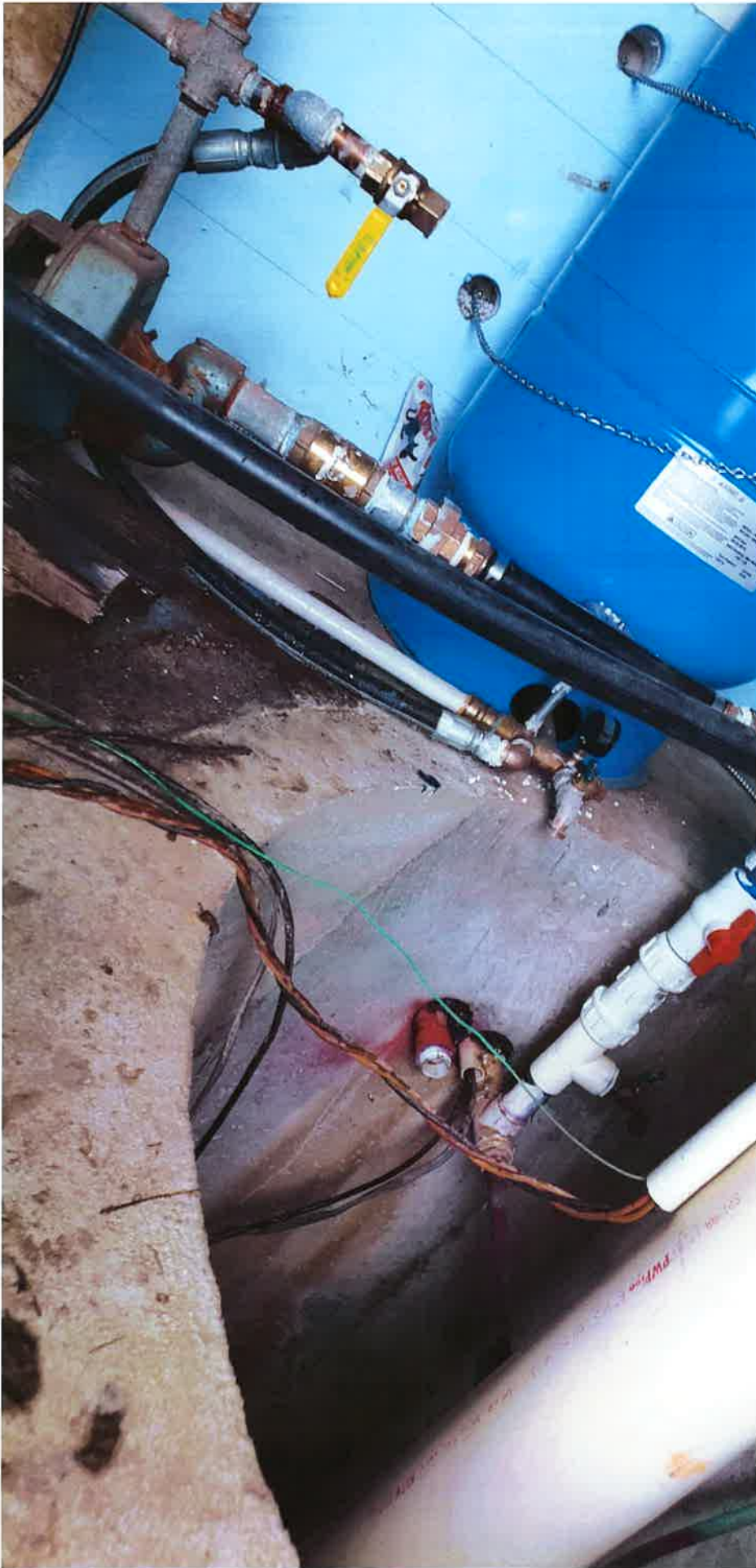
5. Photo showing water line removed from joint water distribution system
