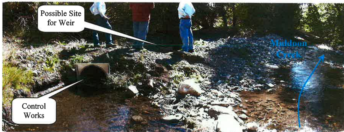
ABOVE: View looking down Muldoon Creek showing the diversion works for the Upper Clark Diversion.
