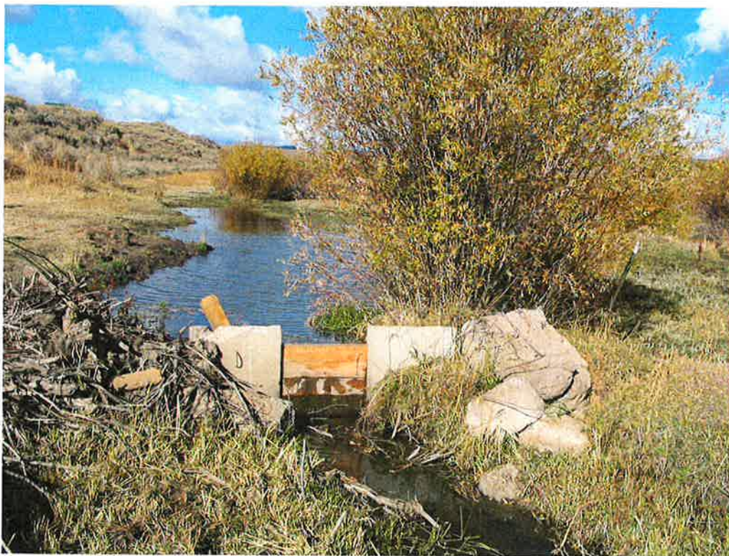
POD #1 – Check structure near POD on Malad River. Photo taken during field exam.
