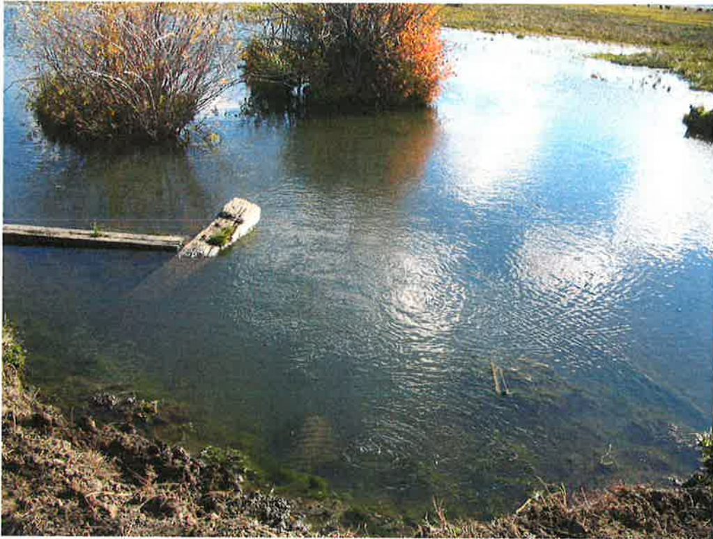
POD #6 – Pipe from outlet gate on east side of pond. Photo taken during field exam.
