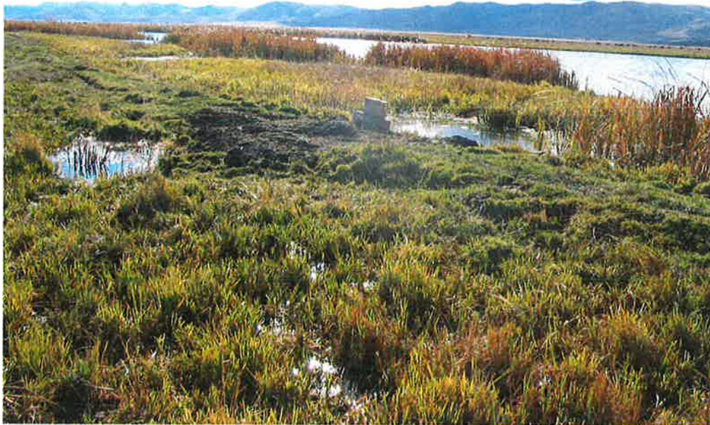
POD #5 – Outlet gate on north side of pond. Photo taken during field exam.
