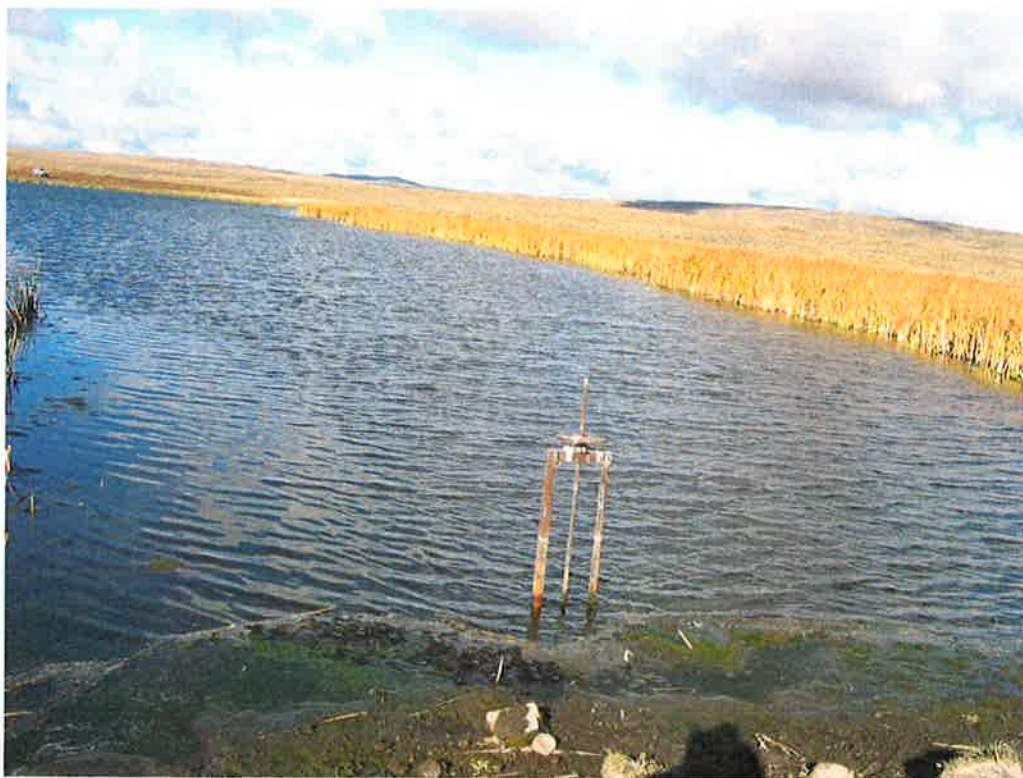
POD #6 – Outlet gate into pipe on east side of pond. Photo taken during field exam.
