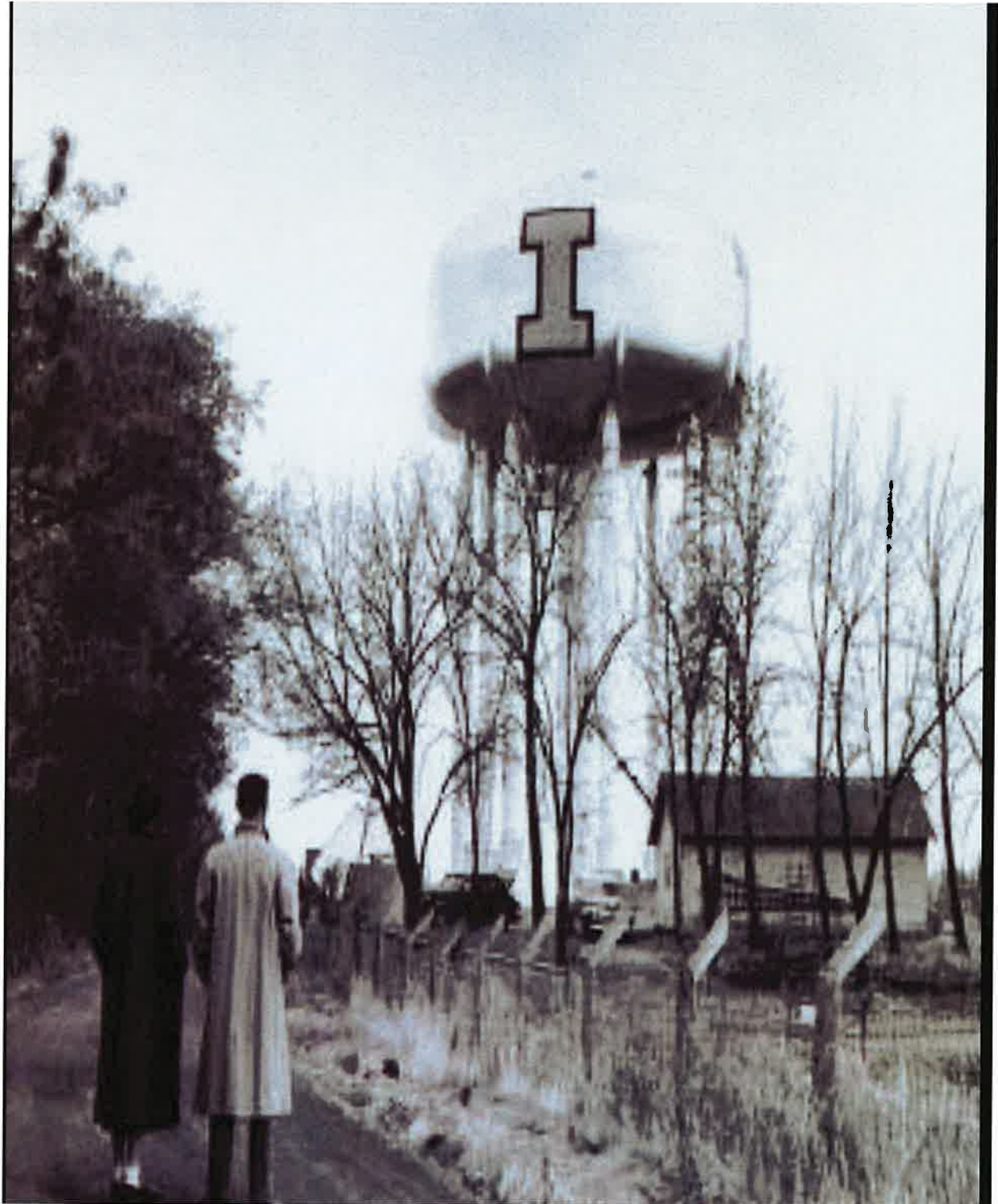
1952 Picture of the 500,000 I-Tank
