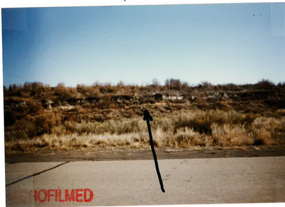
BRALLS FORD DITCH INTO PIPELINE
